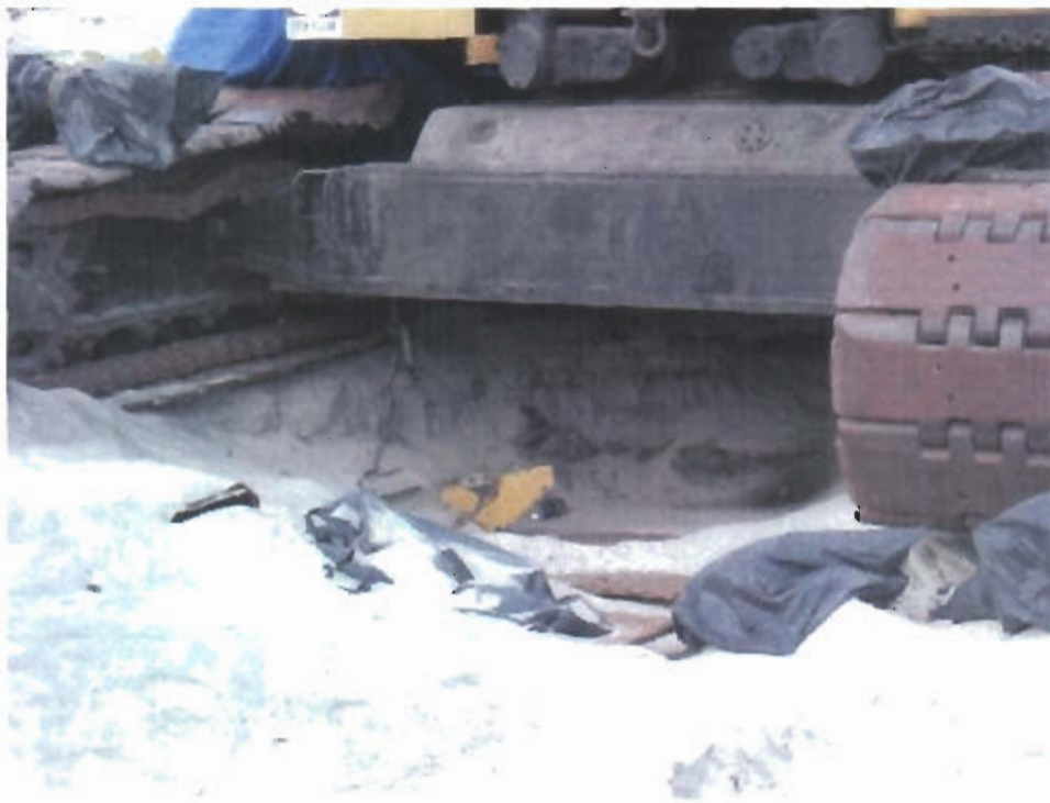
Detail of the pit under the crane, a good illustration that there is absolutely NO barrier or protection from liquid or solid pollutants
