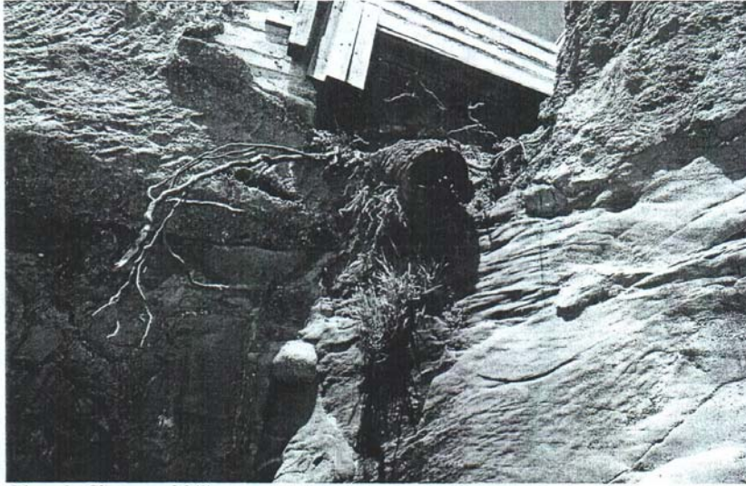
Photo 3: Close-up of failing street-end storm drain.
