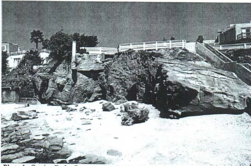
Photo 1: Camino De La Costa street-end and public beach access stairway showing undermined bluff-top public street-end improvements.
