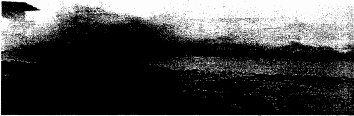
Figure 1. Overtopping of the Pacifica shore protection during an El Nino winter. Note the very dramatic splash. However, the water flowing on Beach Boulevard is only a few inches deep.
