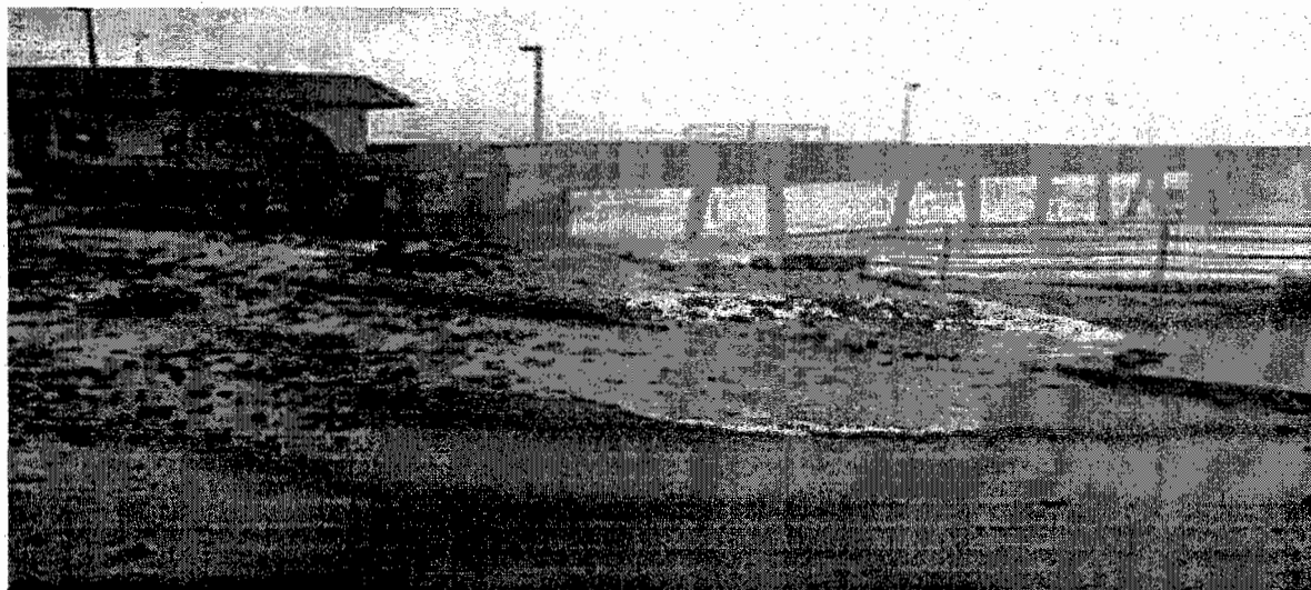
Figure 2. Wave overtopping traveling across Beach Boulevard. Note the water is only a few inches deep and flows down slope along the street drainage path.
