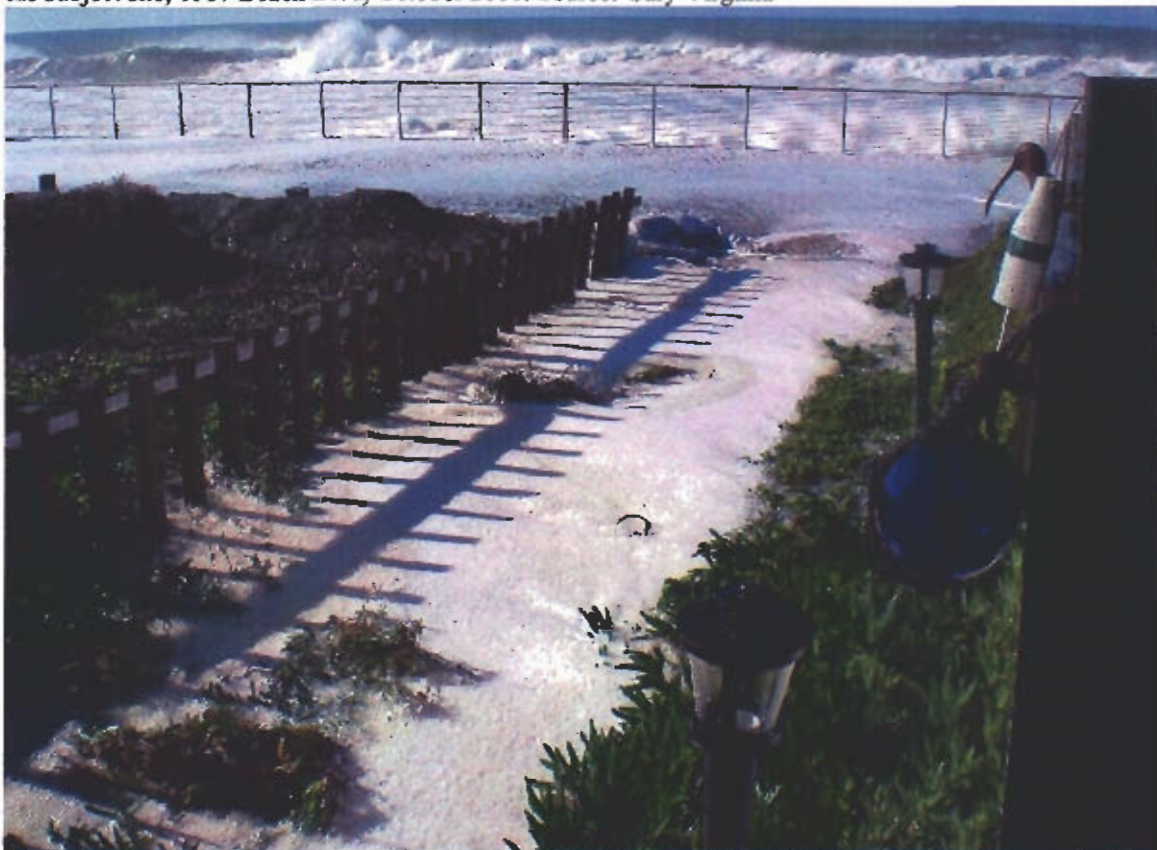
Photo 6 – Wave run-up onto sidewalk and walkway at 1581 Beach Blvd #1, October 2006. Source: G. Virginia
