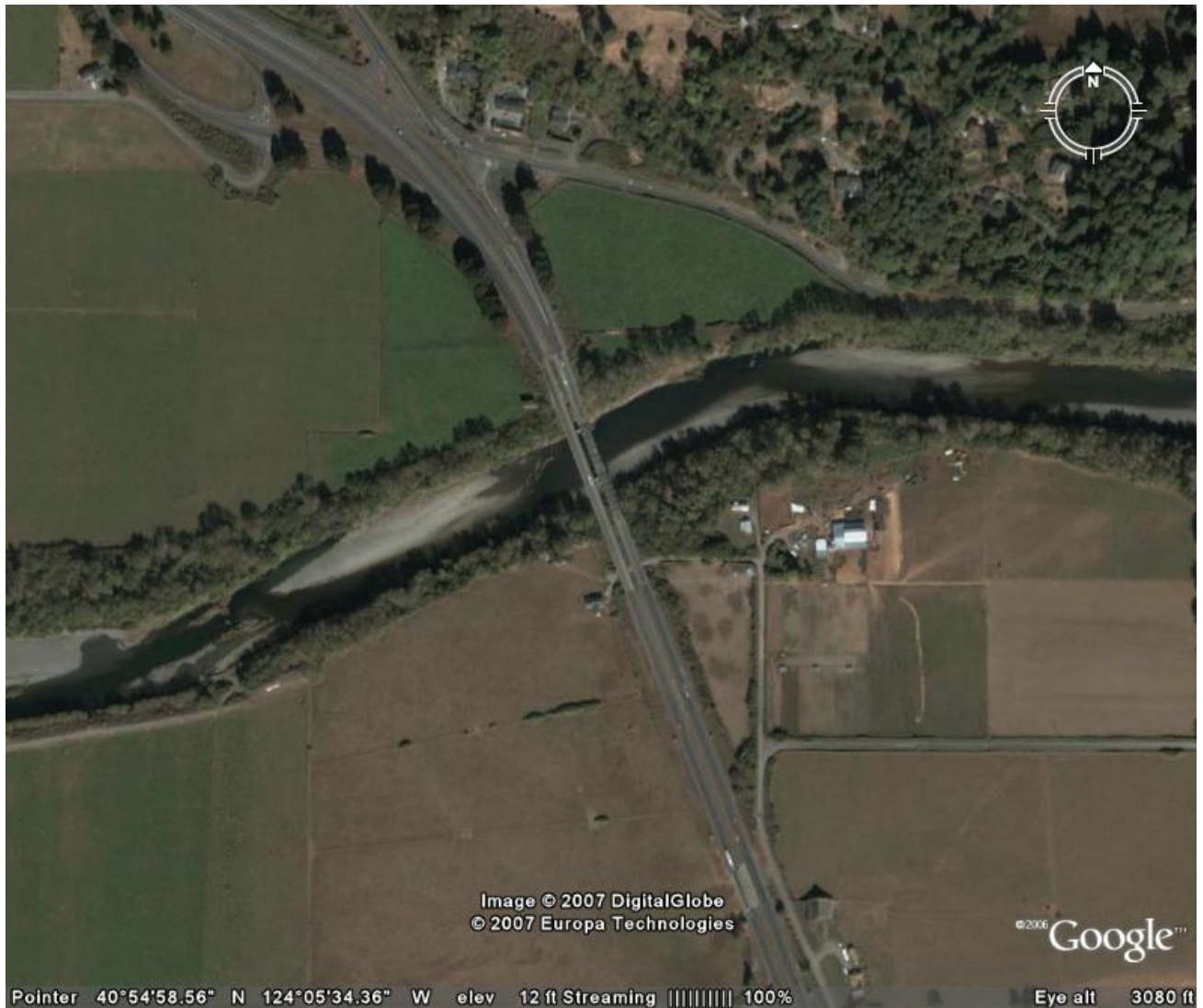
Figure 1. The Mad River Bridges, U.S. Route 101, unincorporated Humboldt County. Source: Google Earth.
