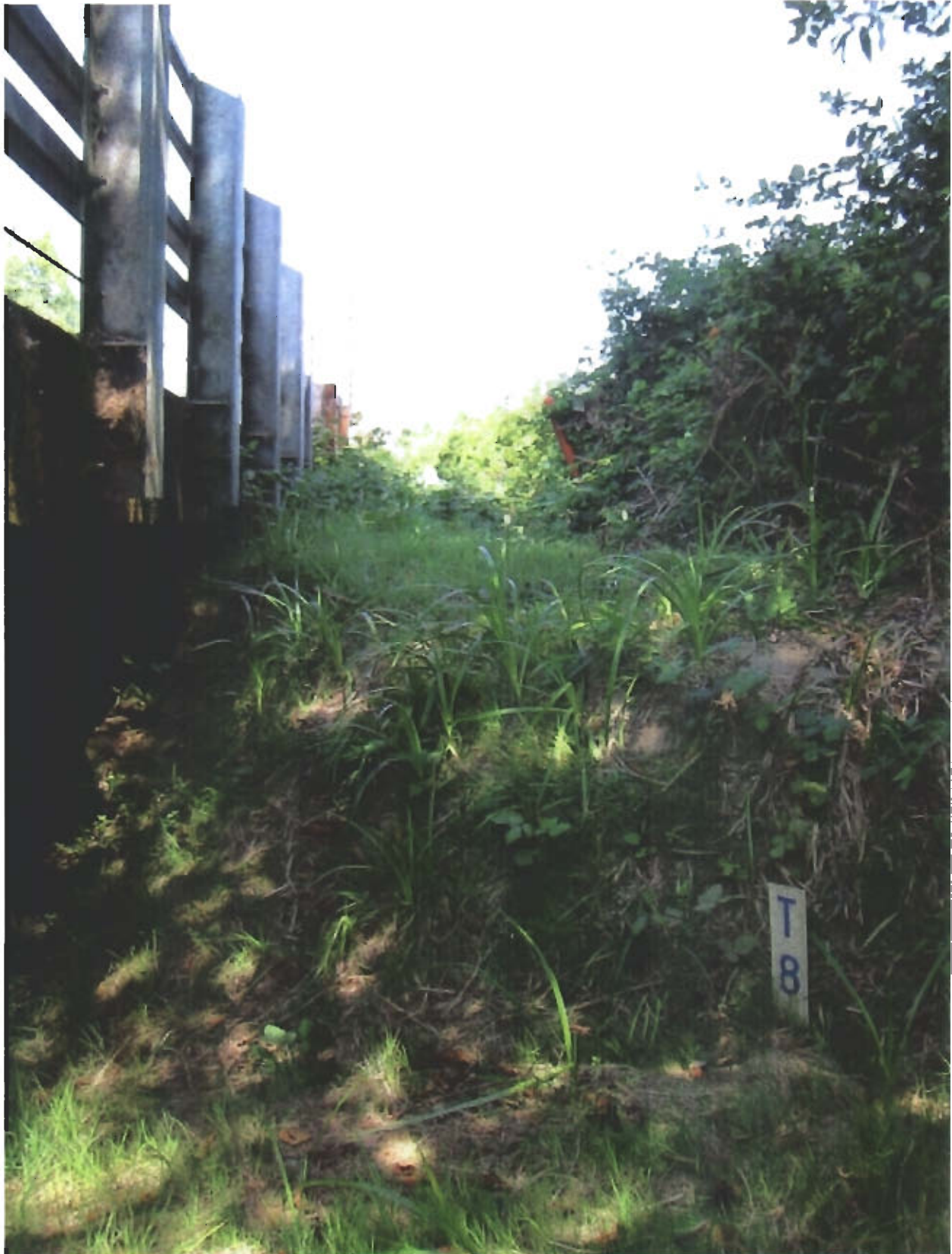
Photo 7: Shows equipment access path from creek channel. Note large amounts of accumulated silt that will be removed to provide equipment access.
