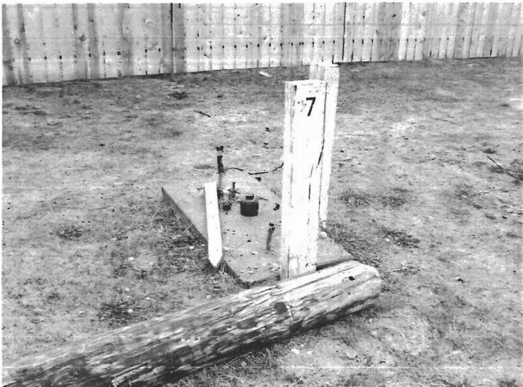
View of Pedestals that need to be replaced.
