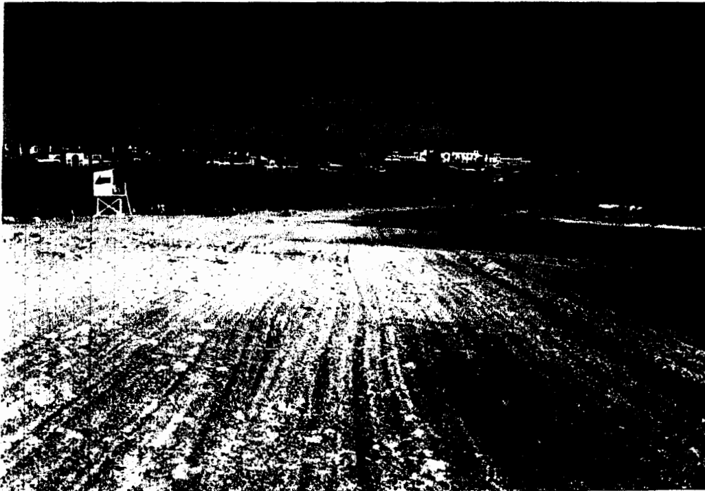
Figure 11. Mechanical Beach Grooming Seaward of The Natural Longshore Beach Berm. August 9th, 2006. Darker areas of beach sand and seaweed beach wrack represent the previous day's high tide line (approximately +6.8 ft MLLW). A grunion run began later in the evening.
