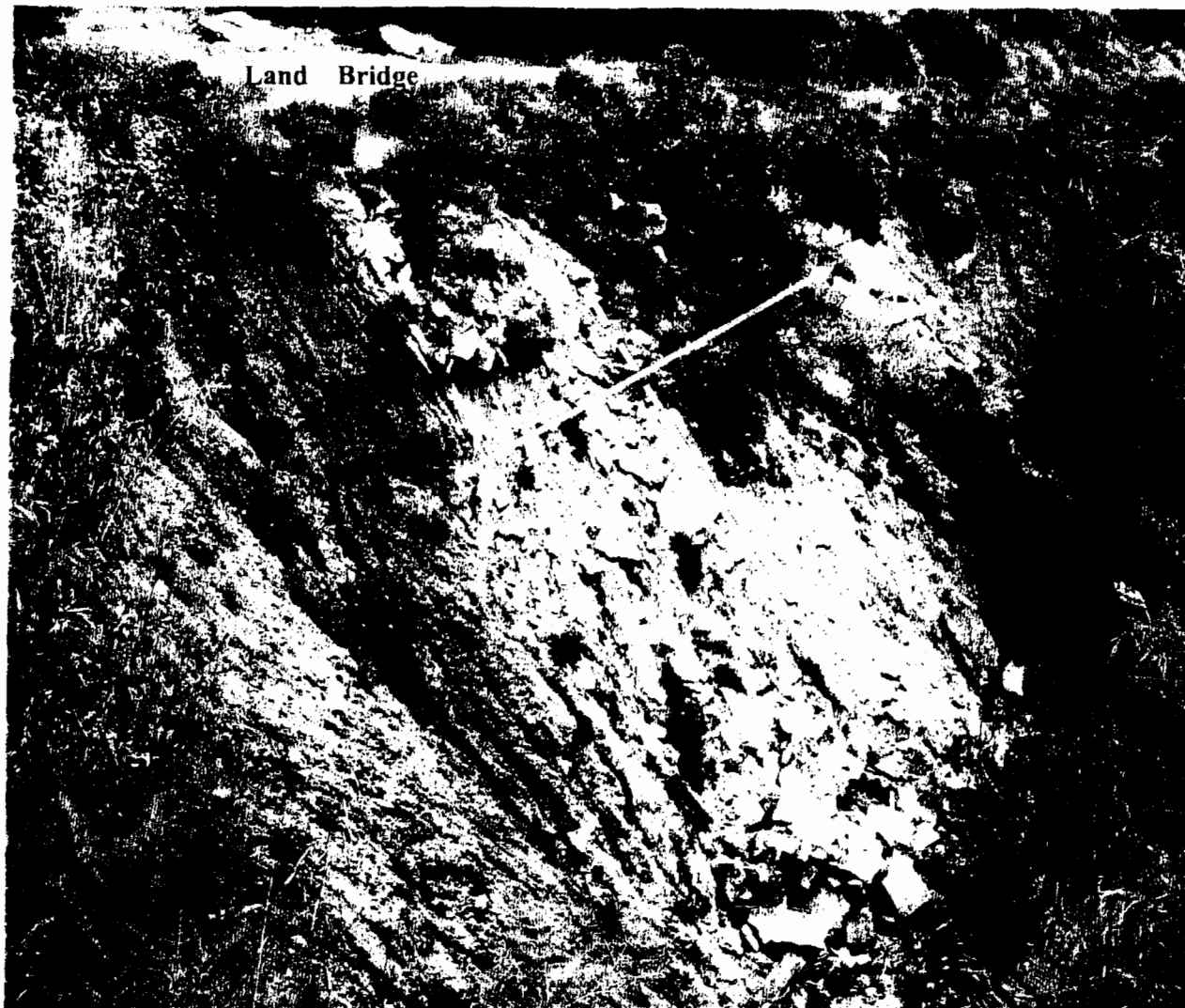
Photo 2 - The steep rubble-strewn slope (red arrows) supporting the narrow "land bridge" is the location of this violation which alleges that "unpermitted fill material was deposited in a riparian area" over this slope (apparently to shore up the land bridge).
