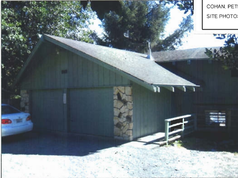
Photo 1. View of the existing garage from the northeast. The existing roofline will be changed to a flat (low-slope) roof with new asphalt composition shingle roofing. This view is not visible from public beaches or trails, but it is visible from Scenic Drive, a public roadway.
