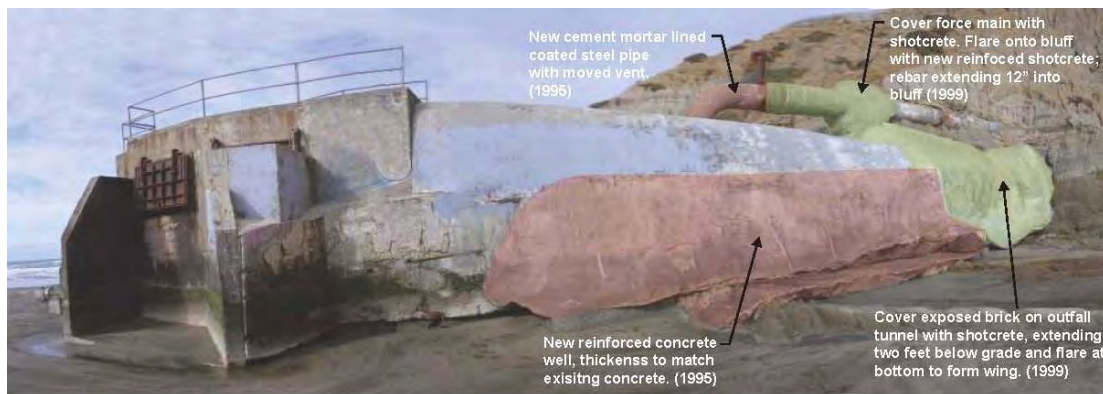
Figure 1. View from the South of 1995 and 1999 Maintenance to Vista Grande Outfall Structure
