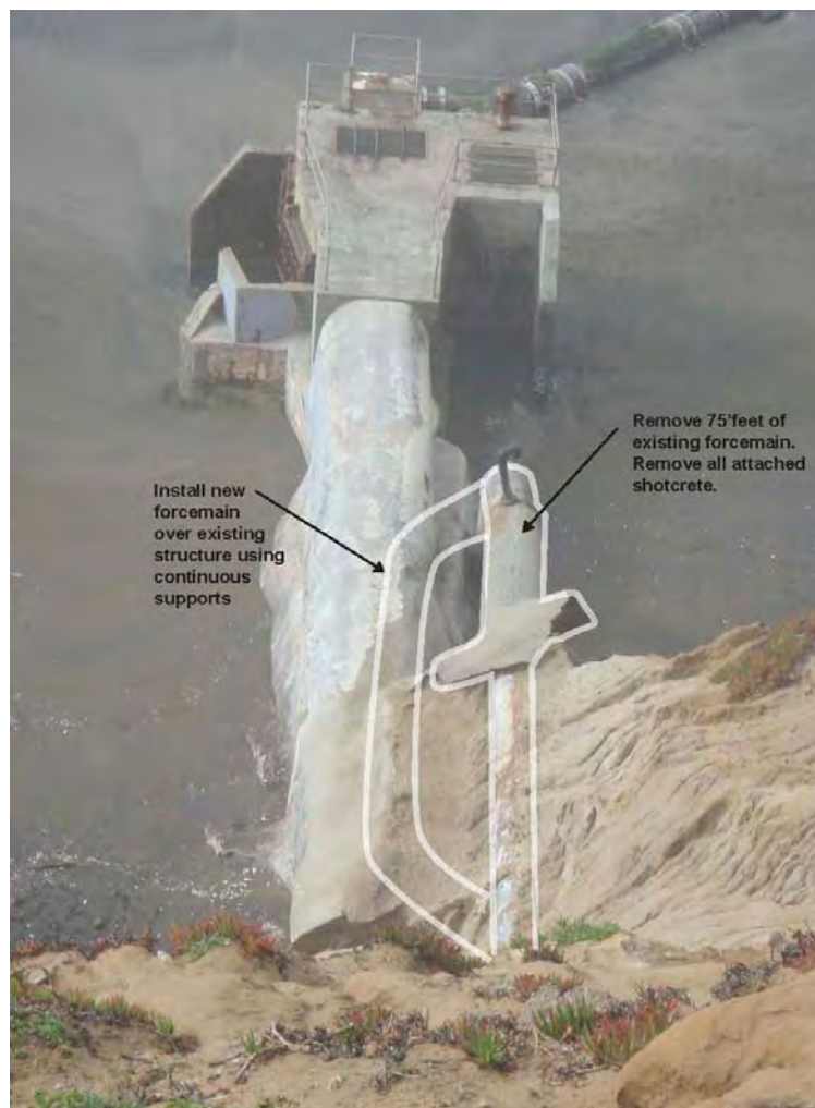
Figure 4. View from Above of Proposed 2010 Maintenance to Vista Grande Outfall Structure
