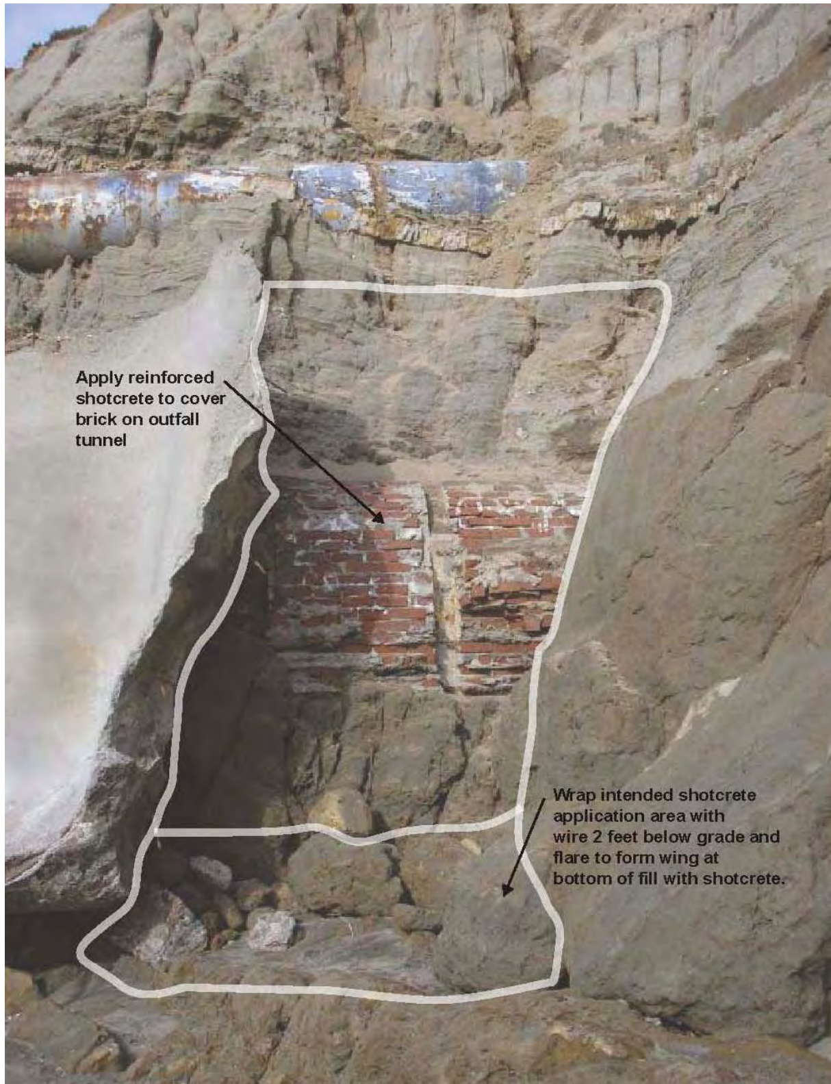
Figure 8. View from the South of Proposed 2010 Maintenance to Vista Grande Outfall Structure
