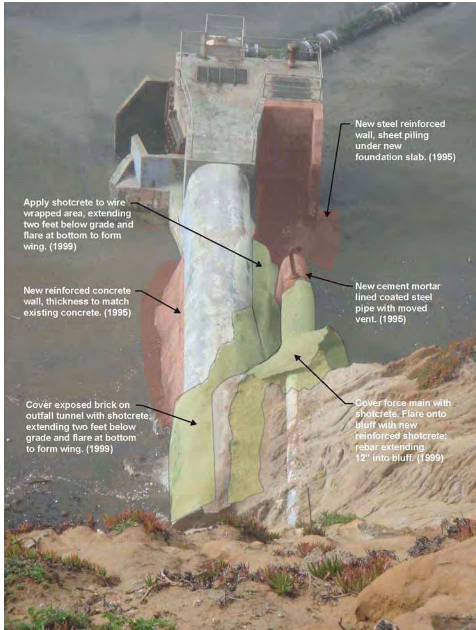
Figure 3. View from Above of 1995 and 1999 Maintenance to Vista Grande Outfall Structure
