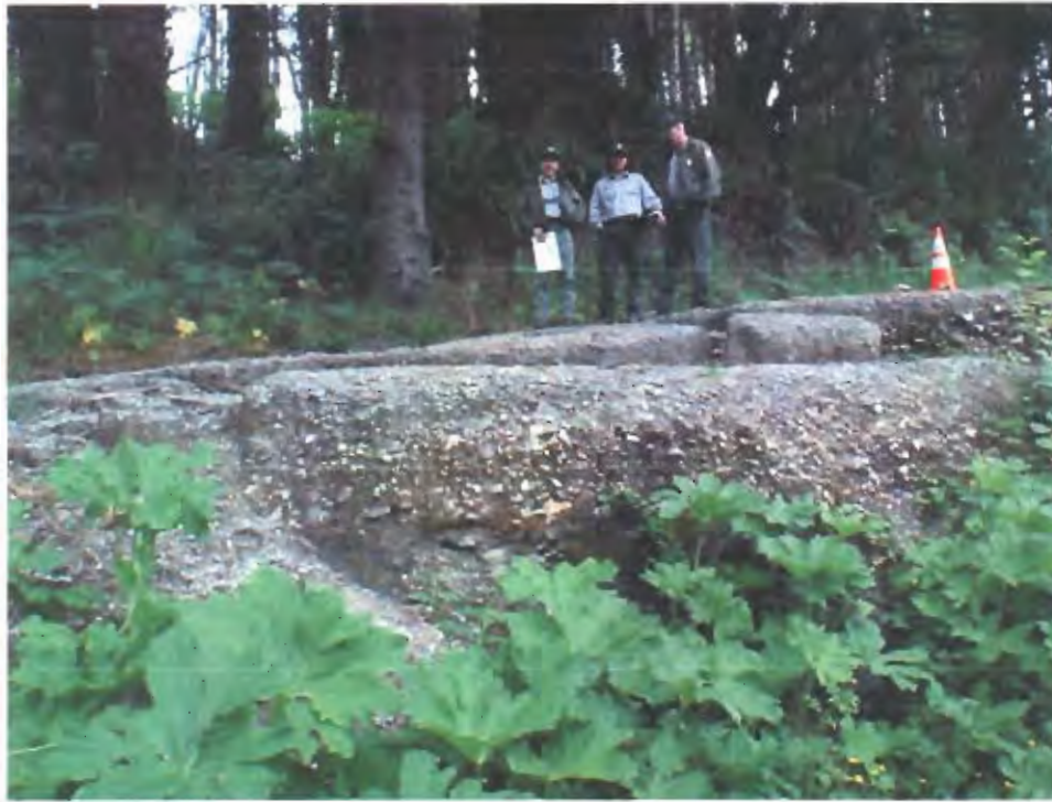
Figure 3. Thick roadway aggregate accumulations within the failed outboard shoulder of the slide closure site.
