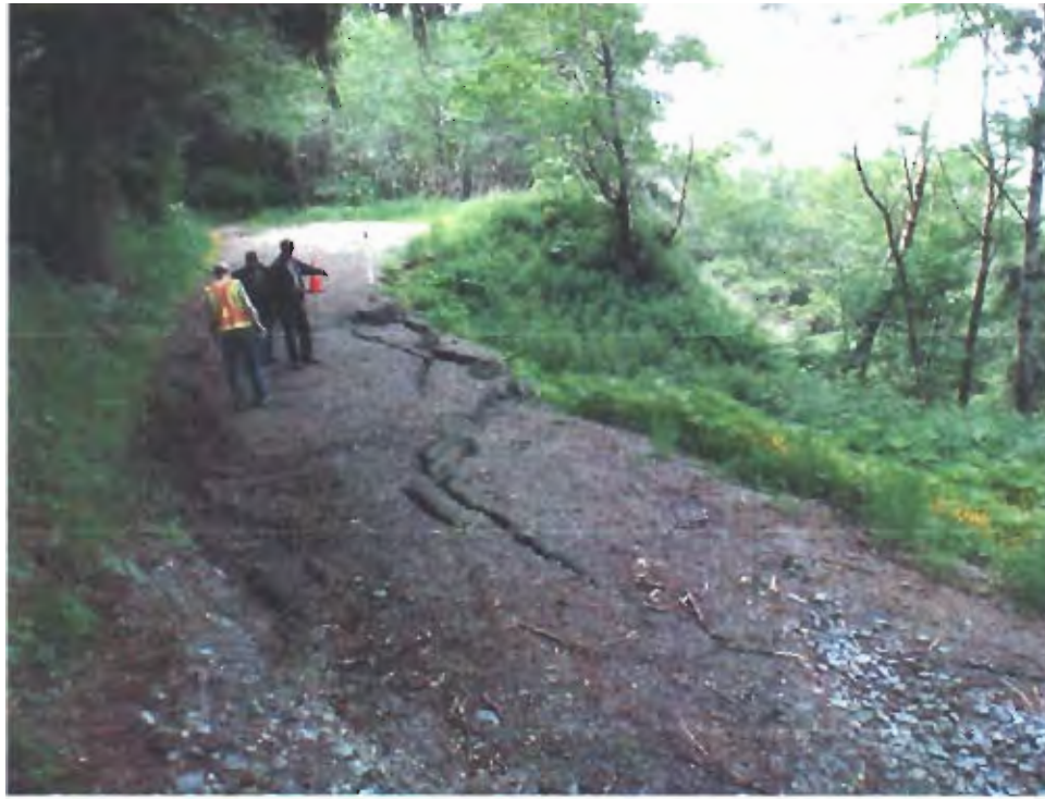
Figure 1. Looking south along the Coastal Drive slide failure. The slide scarp is along the inboard ditchline, with ground movement toward the right and downslope.
