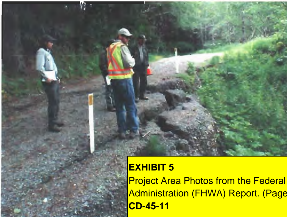
Figure 2. Major cracking (to +4 ft depth) near outboard shoulder at southern limit of the slide. Granular material is from repeated attempts to re-establish grade in recent years.
