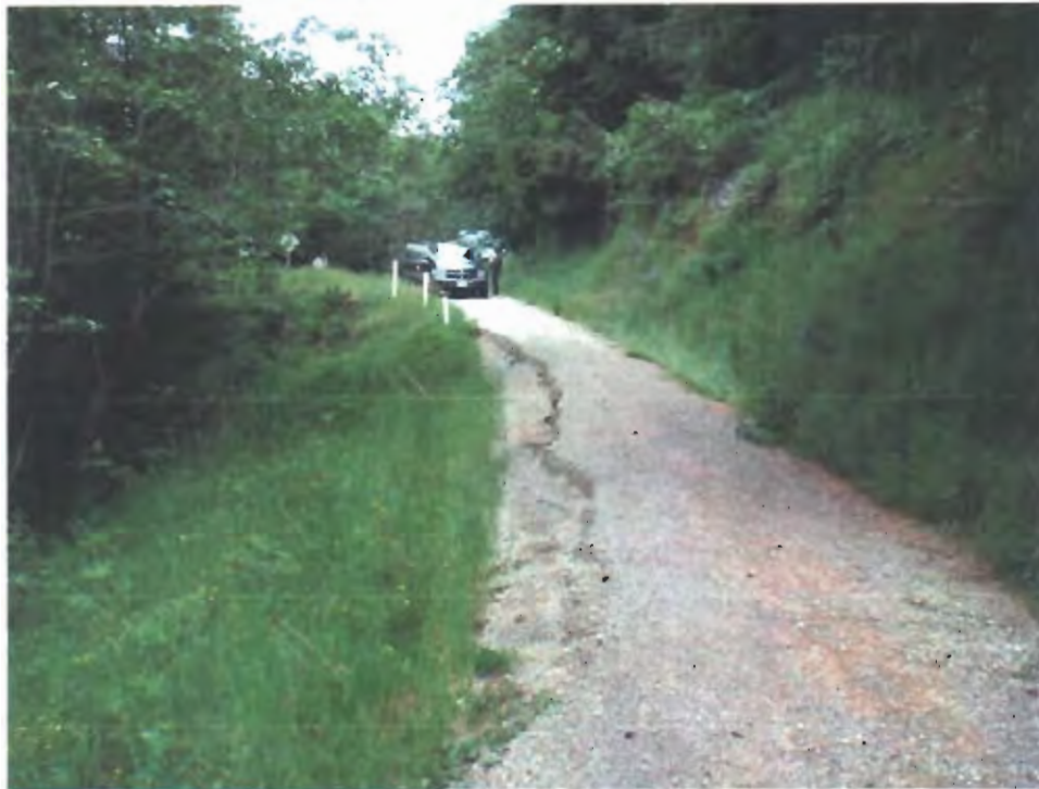
Figure 5. Typical outboard failure requiring a reinforced earth deep patch repair to re-establish the travelway. Simply filling, compacting and regrading these locations will result in continued encroachment of the failure zone across the roadway width.
