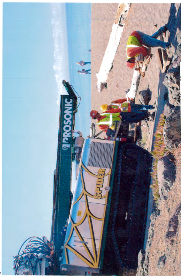
Crew member placing pieces of wood - extending path for prosonic to get onto beach 9-22-10 TD
