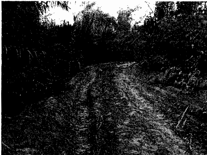
Photo Exhibit E: Represents the Pilot channel after vegetation trimming to delineate the 23-foot work limits and before excavation. Photo taken 11/12/10.
