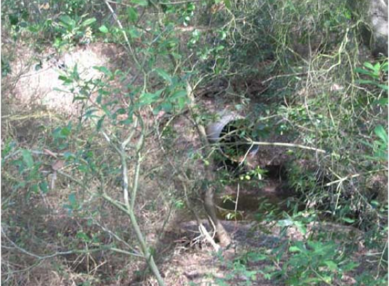
View of existing culvert to be removed
