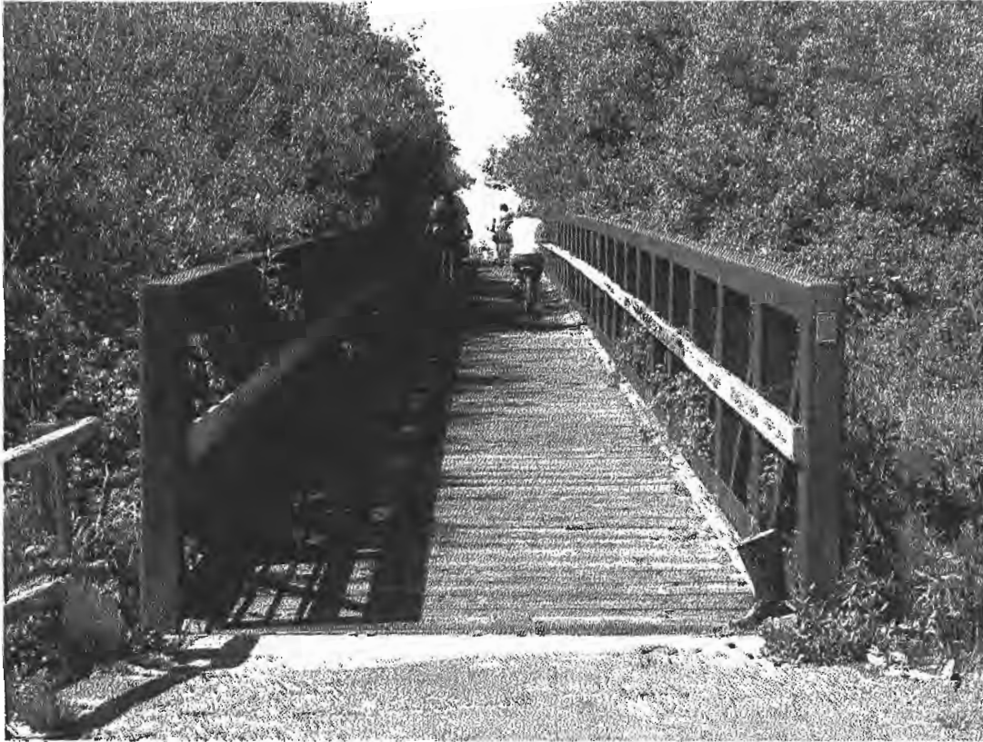
THE NARROWEST BRIDGE ON THE MIDCOAST COASTAL TRAIL, (PILARCITOS CREEK) THE 8' WIDTH PROVIDES JUST ENOUGH ROOM FOR BICYCLES TO PASS WITHOUT HITTING HANDLEBARS. BRIDGE AND TRAIL WIDTH ON THE COASTAL TRAIL THROUGH THE MIDCOAST RANGE FROM 8-12 FEET.
