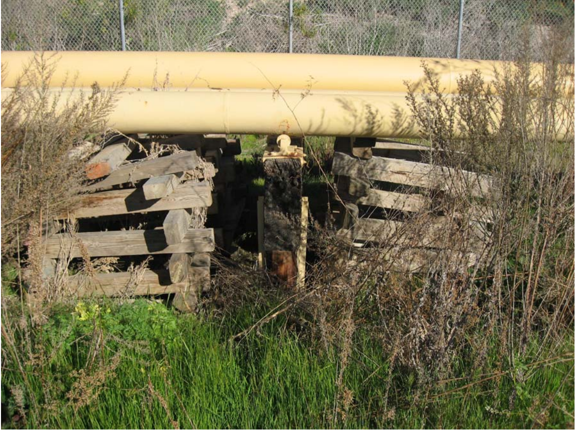
Exhibit 6: Image of existing failing wooden supports.
