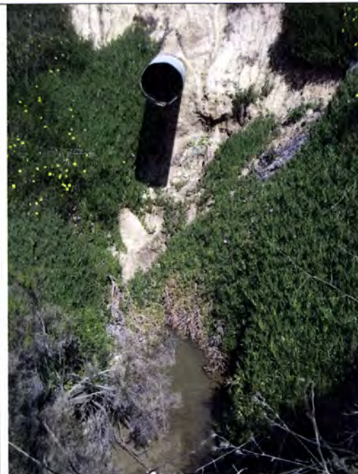
Figure 11. Example of Canyon Area Outfall in Need of Repair
