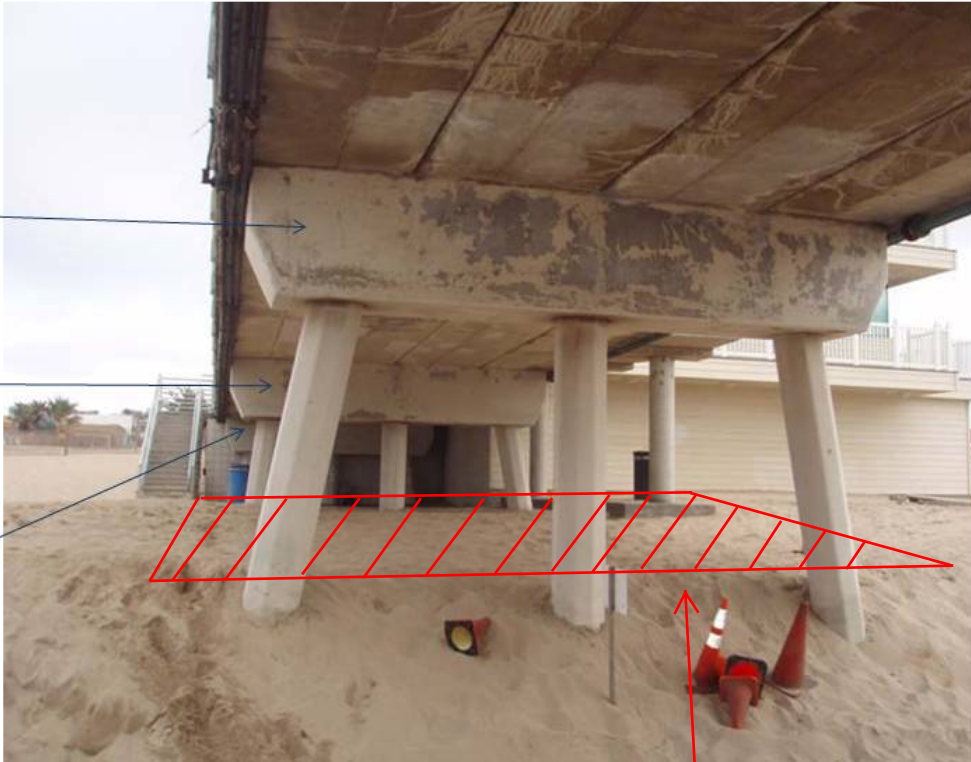
Looking East at Underside of Pier, Bents 5, 4 & 3
