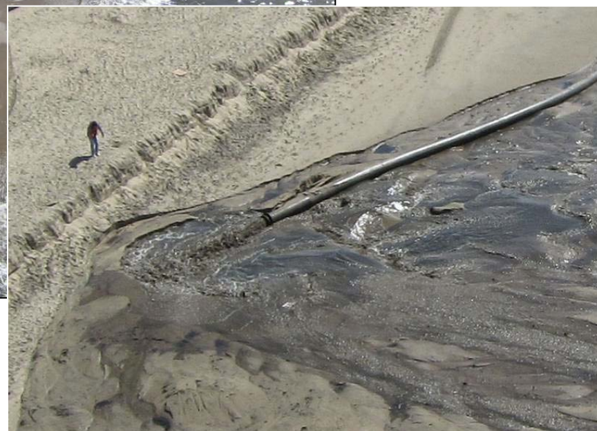
Figure 7. Sand Placement on Beach
