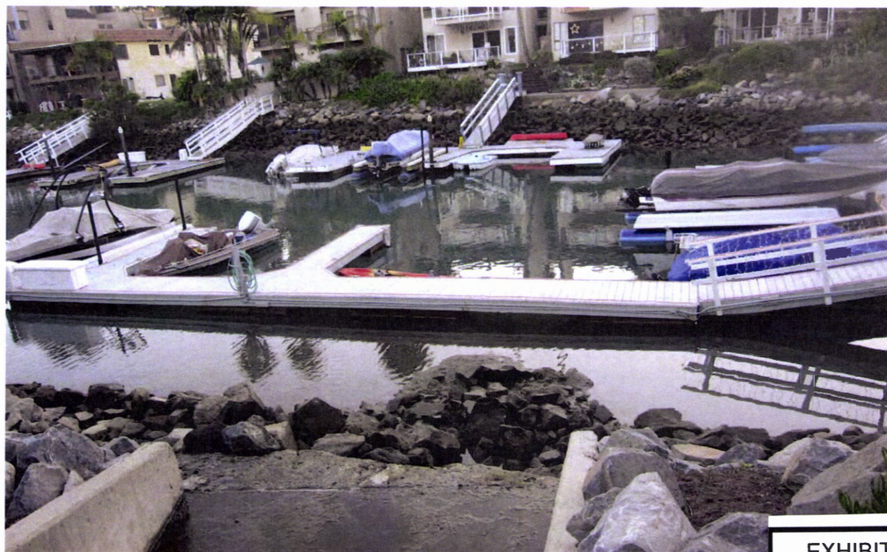
Area of displaced rip rap and sediment.
