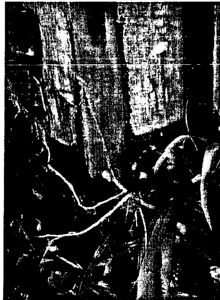
Corner post support columns decayed and suffering exposed water damage on most NW-ernly cabin
