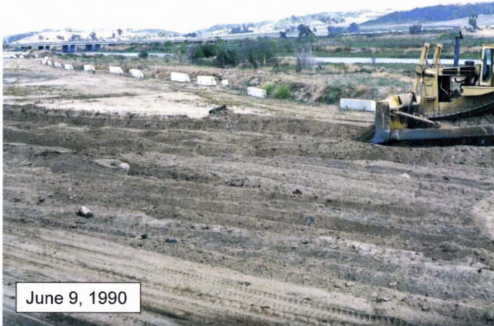
Figure 13. Grading and fill along the south end of the east overflow parking lot roughly in the area where it connects to the south overflow lot.
