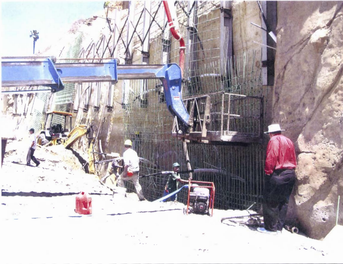
Figure 15: Base of seawall under construction
