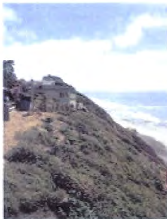
MARCH 2003 NOTE HYDROSEEDING SLOPE
