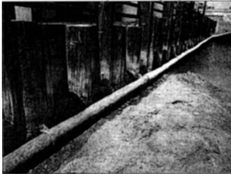
Poche Clean Beach Project - Discharge Pipe Along Bulkhead
