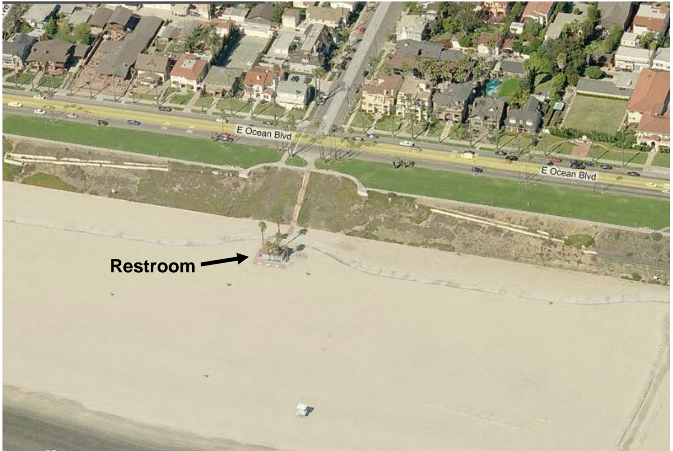
Project Site: Bluff Park Beach, at the terminus of Coronado Avenue, Long Beach.
