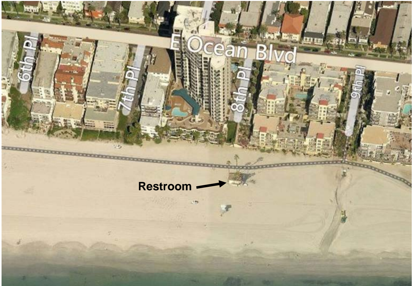
Project Site: Alamitos Beach, at the terminus of 8 th Place, Long Beach.
