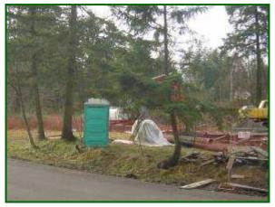
Figure 1. Improper storage of materials.
