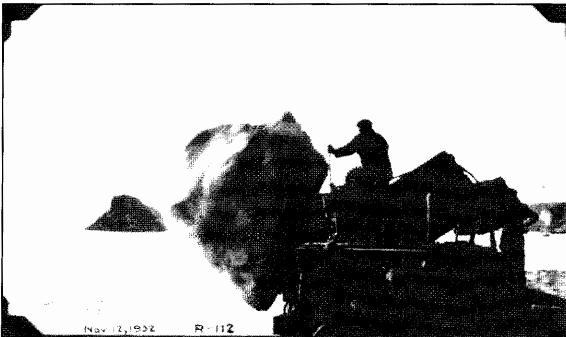
Figure 5: Placement of Individual Large Armor Stone in November 1932
