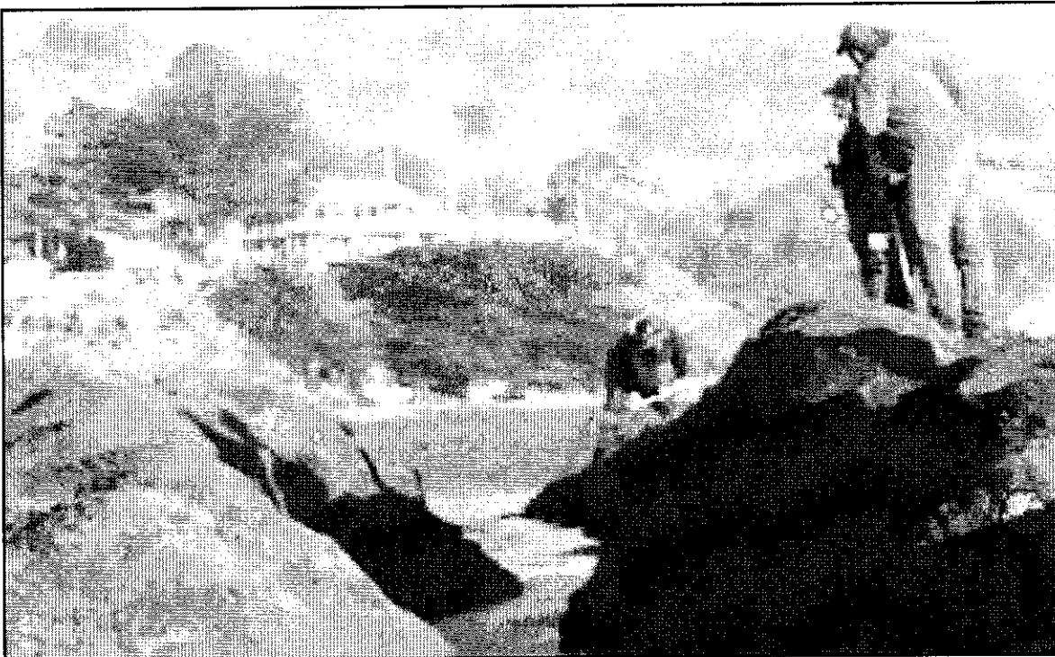
Figure 10: Using Shovels to Open the Russian River Sandbar in 2005
