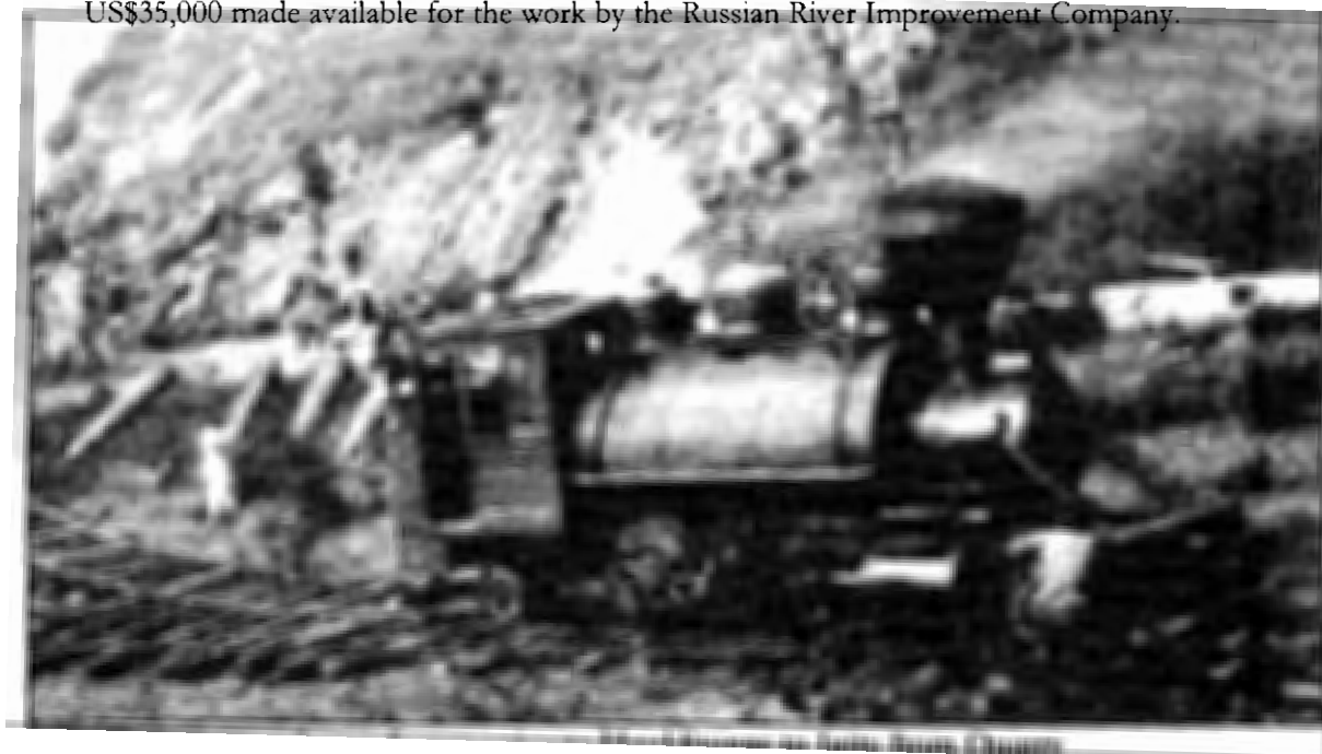
Figure 3: Narrow Gauge Locomotive to Haul Stones to Jetty from Quarry
