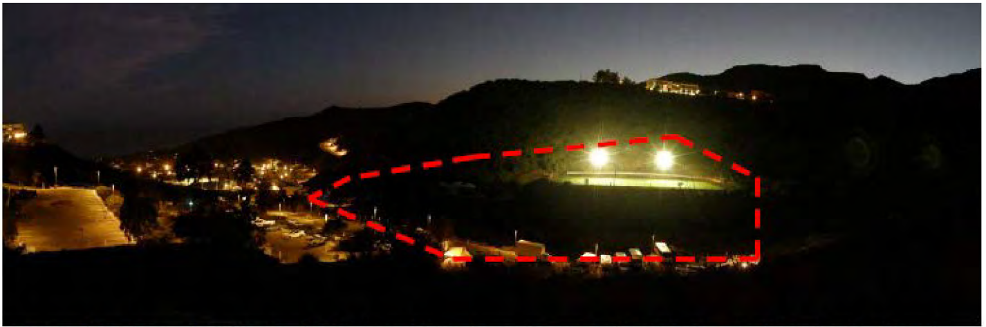
Figure 18: Receptor Site D, Nighttime View (component site 5 indicated by dashed box)
