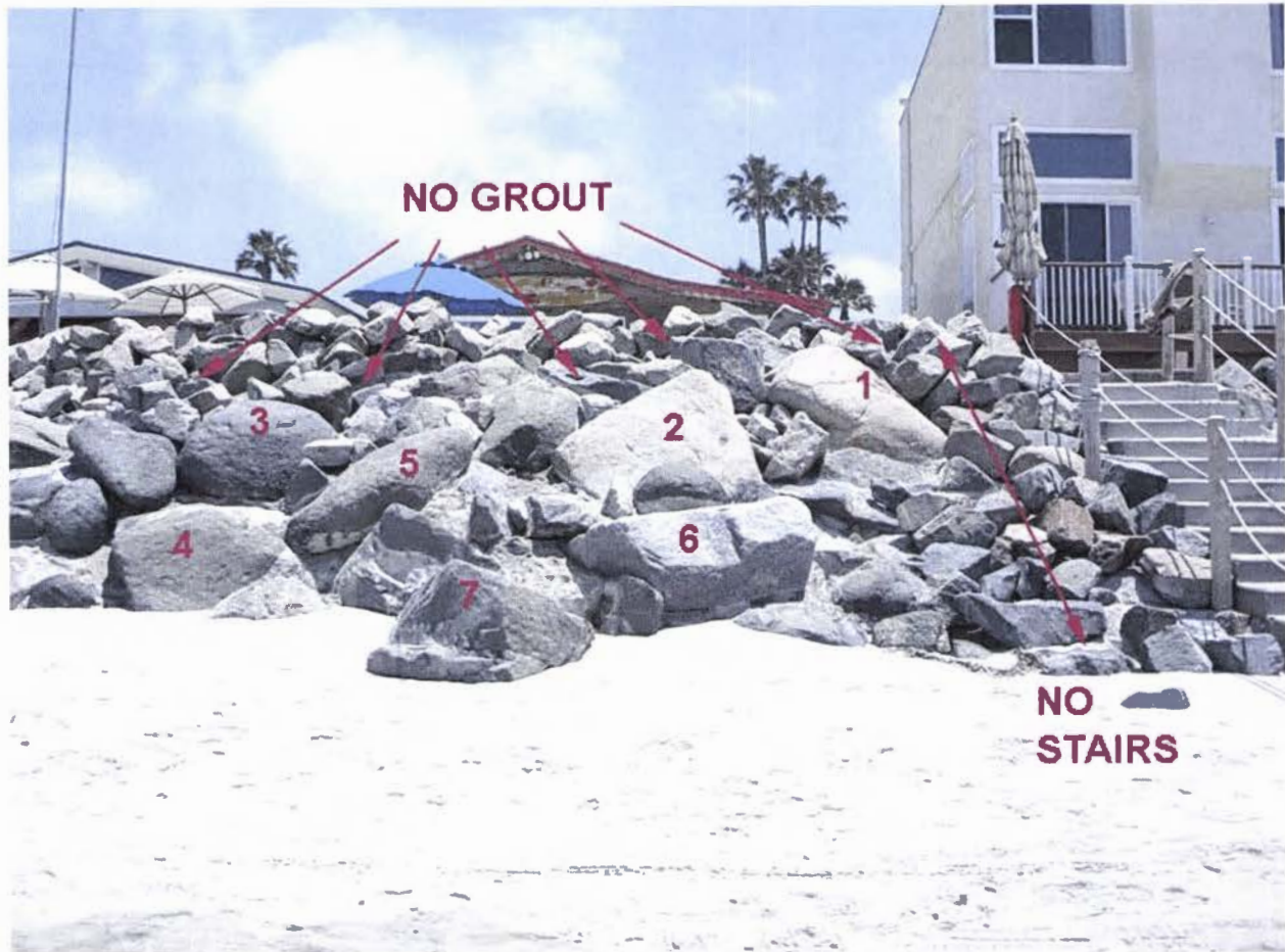
Figure 2. Subject revetment after the maintenance. Note the positions of the numbered rocks has not change.
