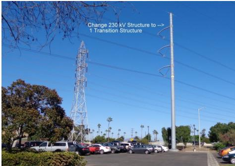
Figure 6 Proposed Location of Transition Structure with 1,000 feet of Underground Transmission Cable
