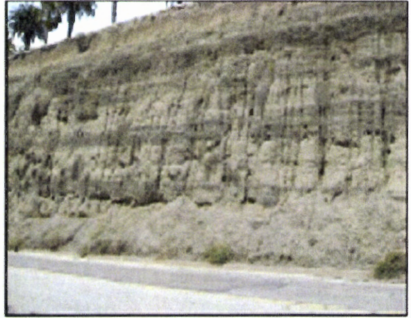
Erosion Gullies in Slope
