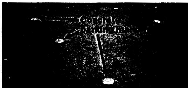
Figure 8-16--Concrete markers are used to delineate unpaved parking spaces in some areas of the country.
