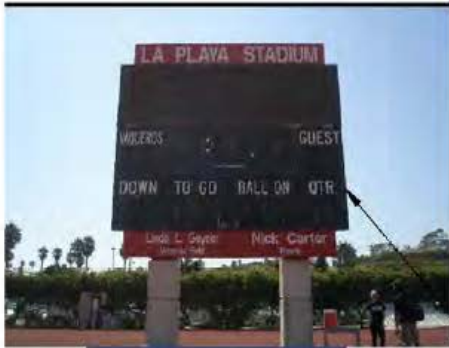
FRONT OF EXISTING SCOREBOARD WITH SCREEN HEDGE AT PARKING AREA TO WEST BEYOND
