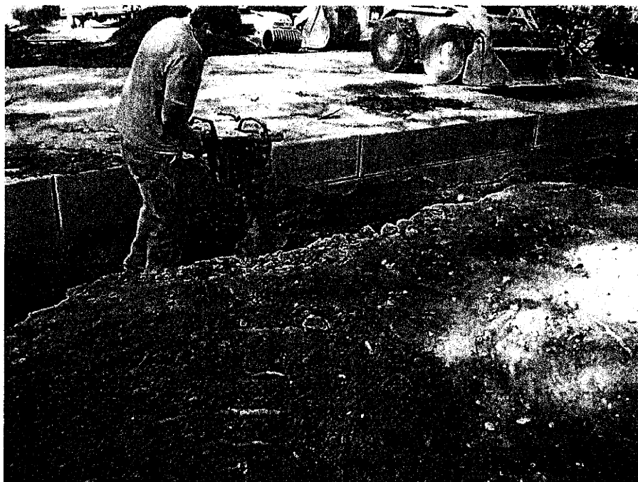
BACKFILLING CULVERT
