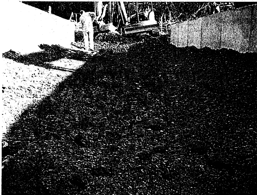
BACKFILLING INVERT WITH RIVER RUN
