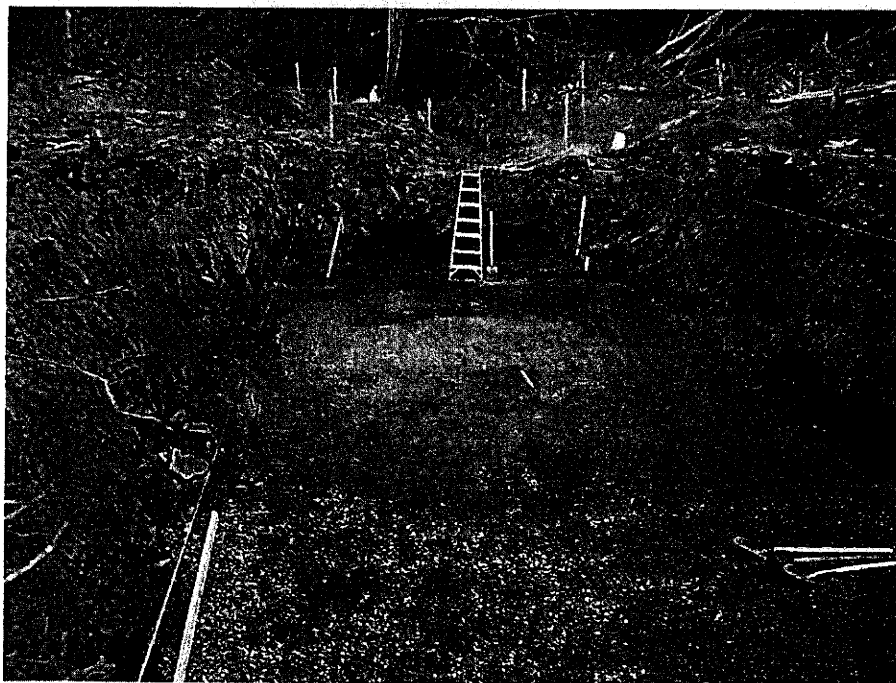
PREPARING CULVERT BEDDING
