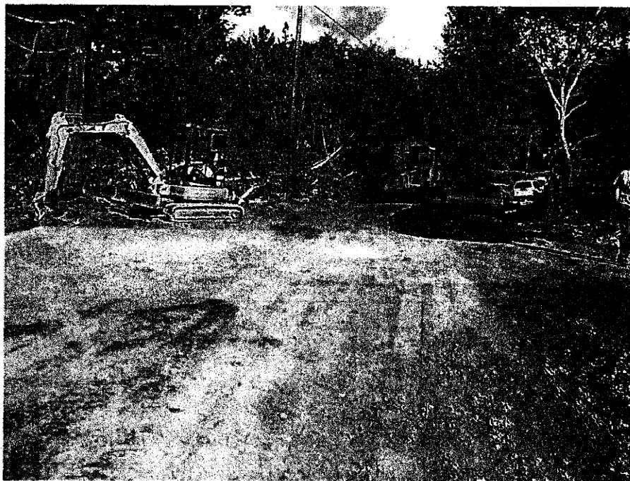
PLACING AGGREGATE BASE
