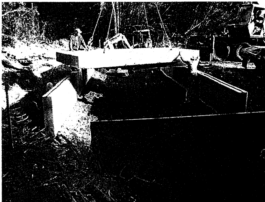
PLACING CULVERT TOP
