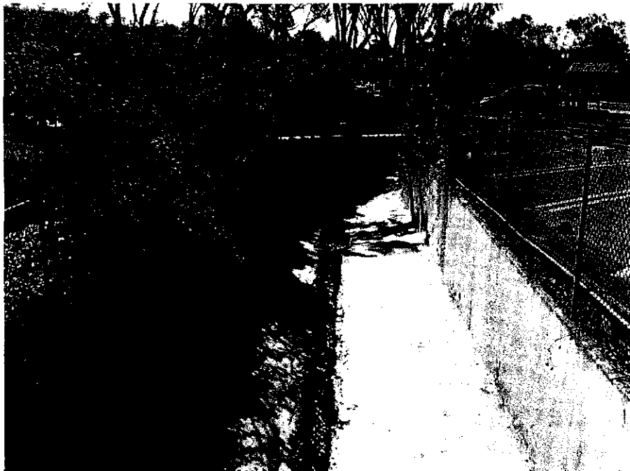
Figure 6. Looking downstream toward Forest Avenue from maintenance yard bridge (open 15' x 6' rectangular RC channel).
