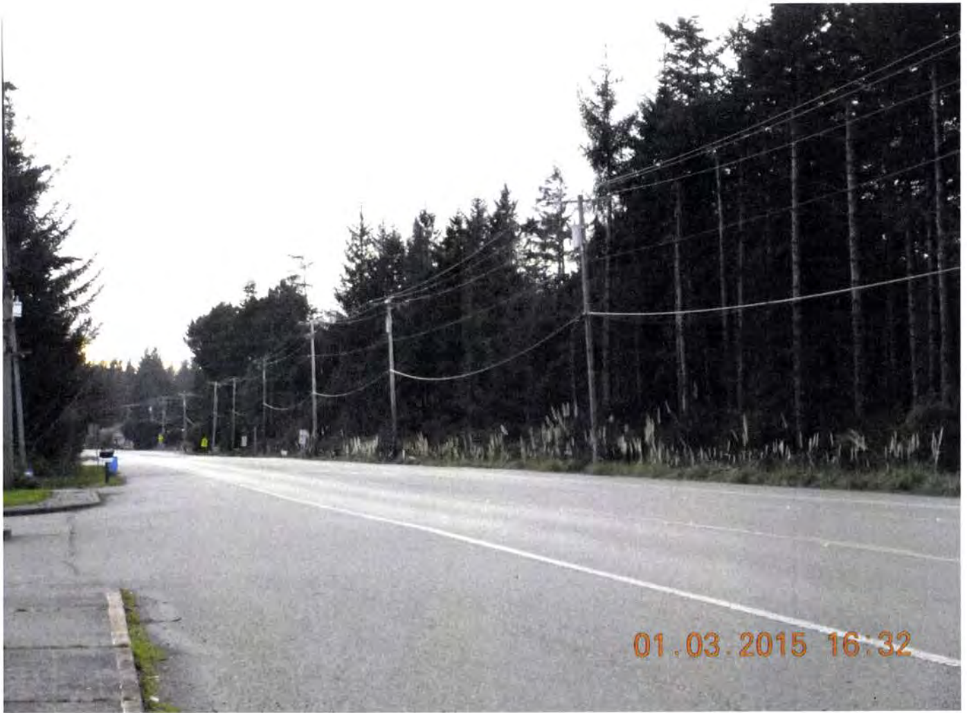
Photo shows Lake Earl road frontage at the mitigation site. Invasive Pampas Grass is out of control and invading the mitigation area from this vector. Invasive vegetation is easily accessed here and should be removed.
