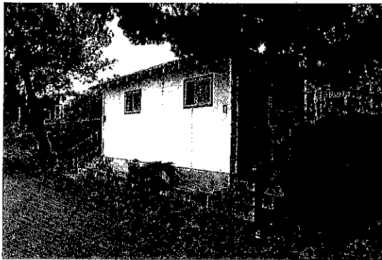
Figure 36. Northeast and northwest facades Source: Page & Turnbull, 2013
