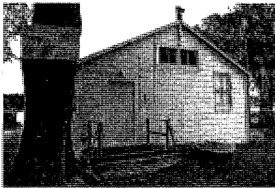
Figure 39. Southeast façade. Source: Page & Turnbull, 2013
