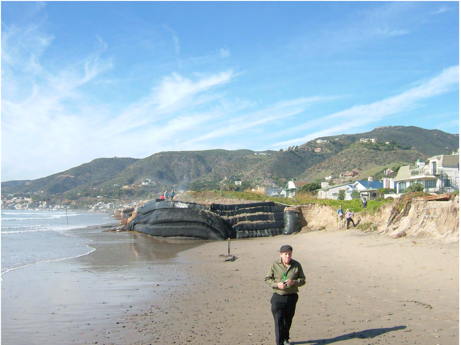
Effects of Seawall on the Width of Broad Beach (Fixing the Back of the Beach)
