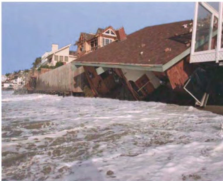
Photo 3. Storm Damage Wave action in the 1997-1998 El Nino led to major structural damage to one home on Broad Beach (Source: Norton Karno, 2/98)
