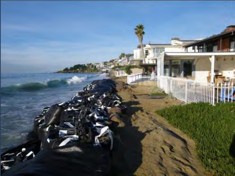
West Broad Beach Sandbagging- Pre revetment
