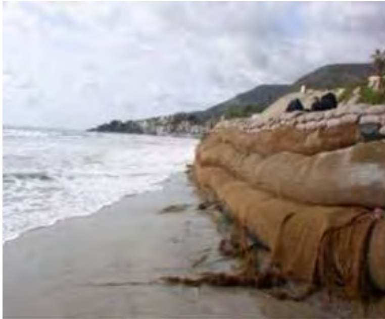
Photo 4. Geotextile Bags 2008-2009
