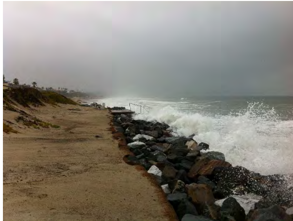
Photo 9. Wave Run Up March 2014 Overtopping of the revetment occurred during storm wave run up on March 3, 2014 during an estimated 5-ft tide.
