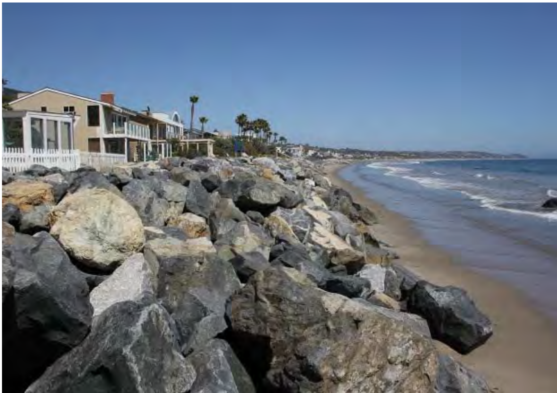
Photo 12. Revetment Toe
