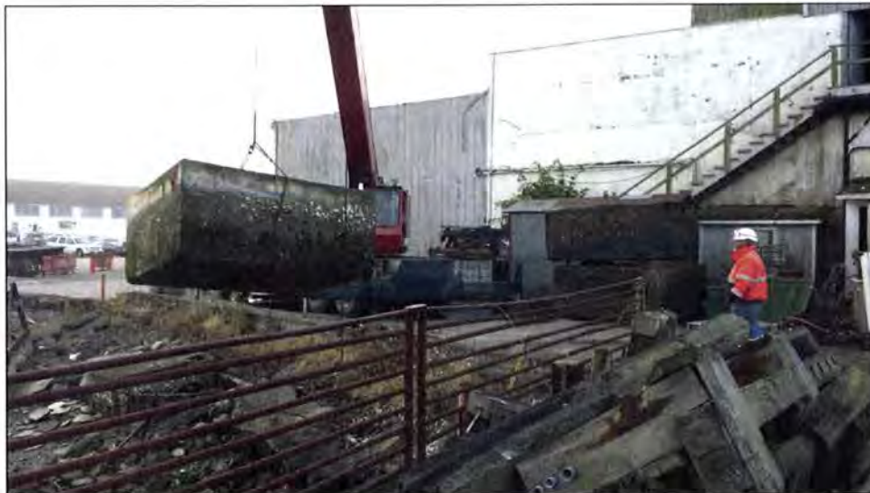
Photo 16. Concrete Float Hoisted Ashore (Photograph Courtesy of Stephen Kullmann)
