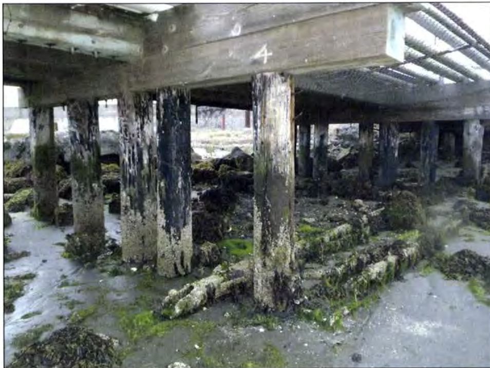
Photo 6. Pile 4S, Scheduled for Replacement in 2015
