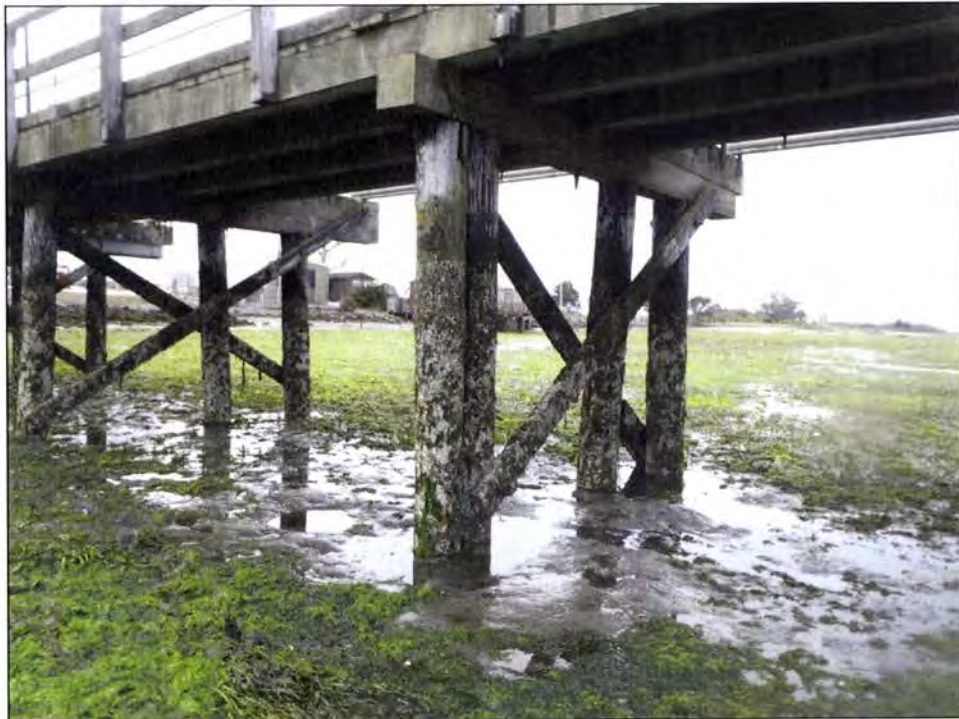
Photo 8. Pile 10N, Scheduled for Replacement in 2015
