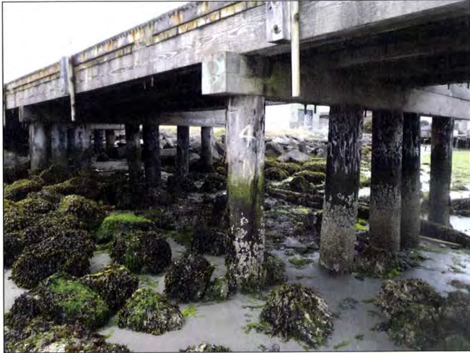
Photo 7. Pile 4N, Scheduled for Replacement in 2015
