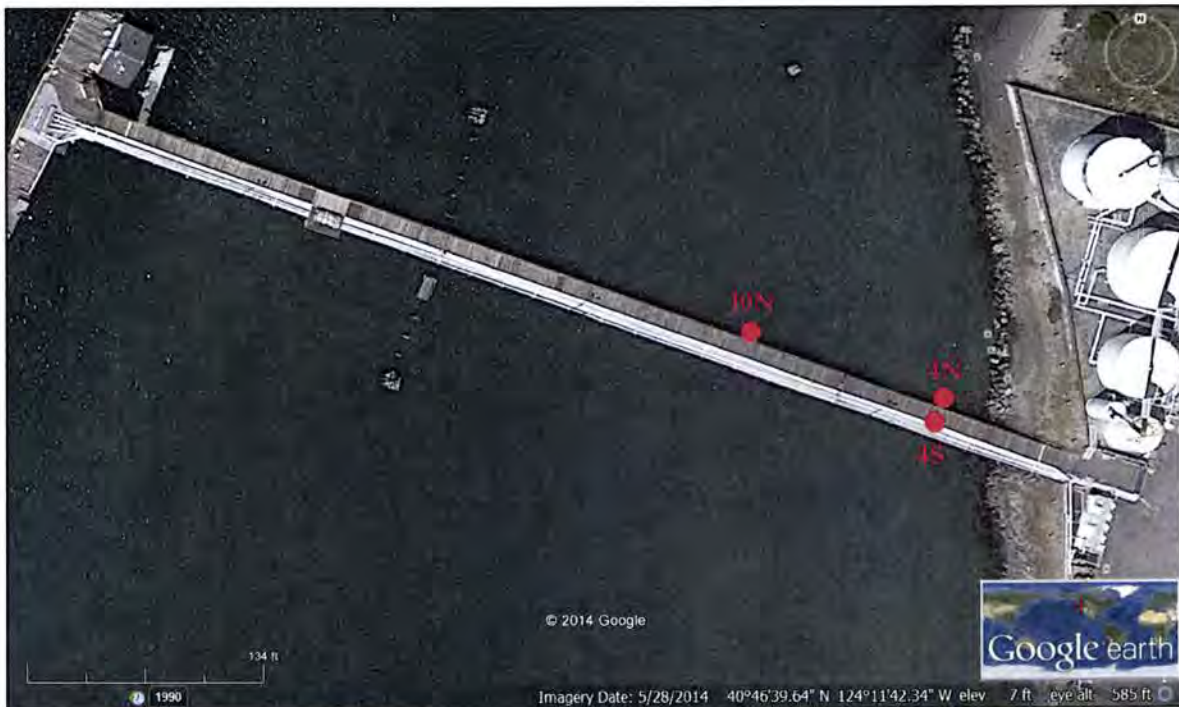
Figure 5. Location of Trestle Piles Scheduled for Removal in 2015
