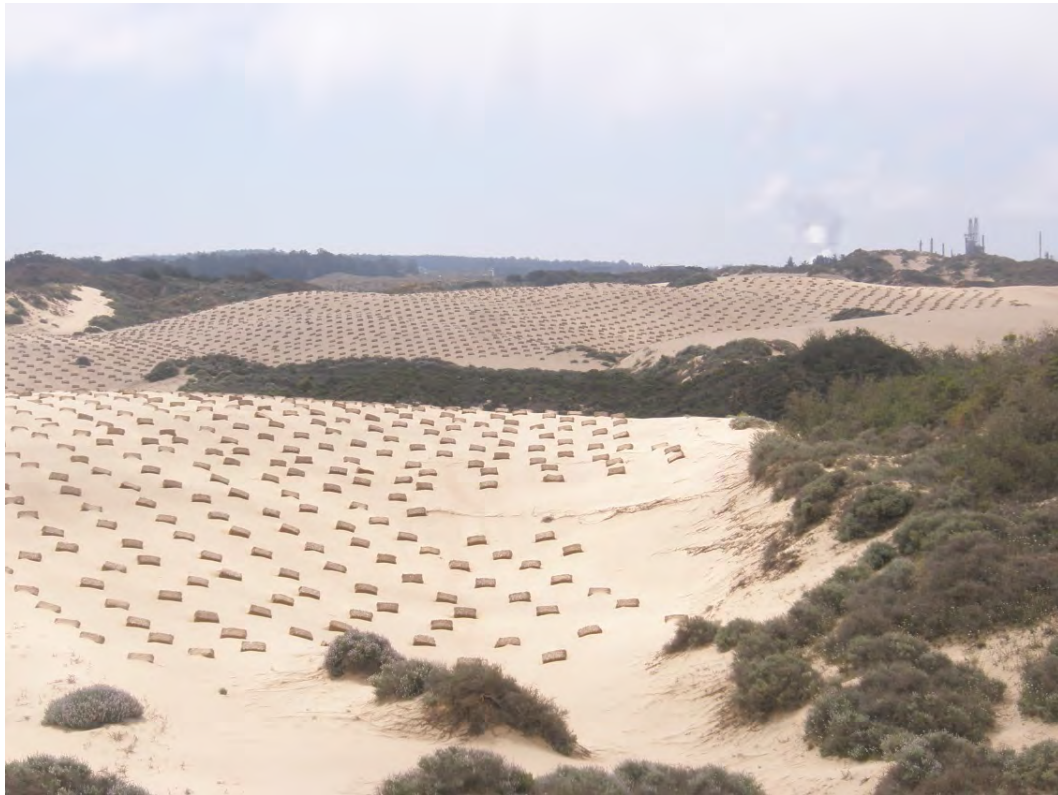
Figure 6: Oceano Dunes Straw Bale Mitigation Treatment
