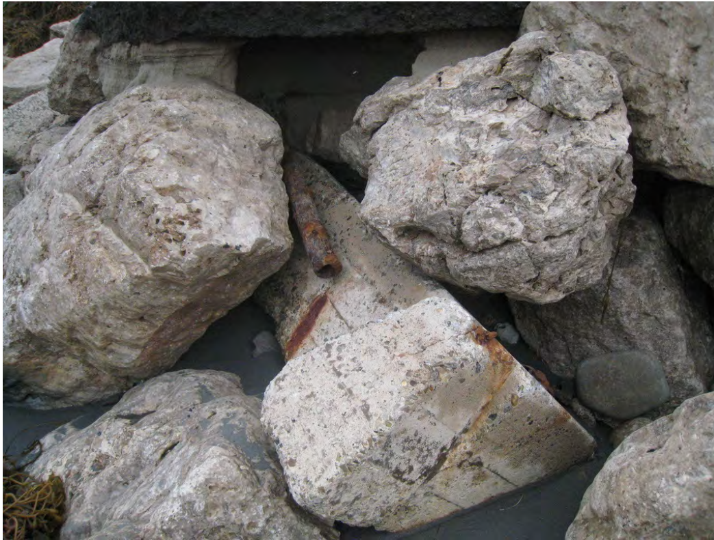
Concrete, rusty pipe, and rebar in Goleta Beach Park west end revetment.
