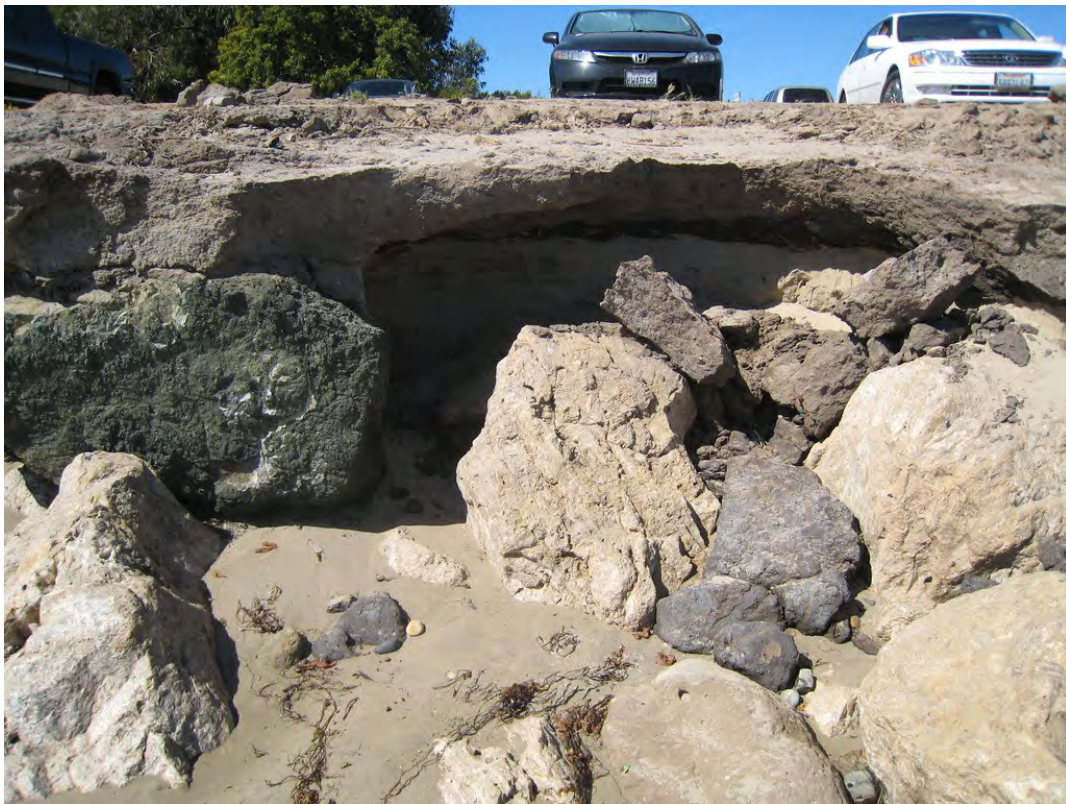
Large pieces of asphalt fall from parking lot 7 into the surf zone.
