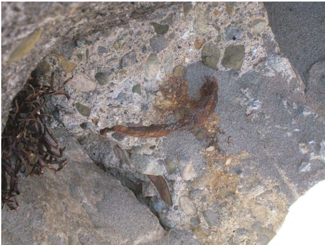
Dangerous rebar in the Goleta Beach Park west end revetment.
