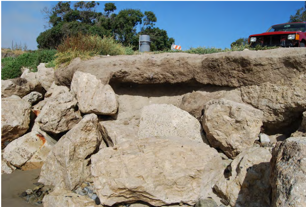
Haphazard revetment fails to protect parking lot 7. Note large concrete blocks at lower left and center of photo.
