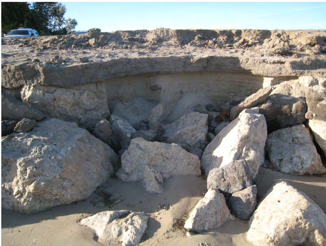
Parking lot undermined at gap in west-end revetment.
