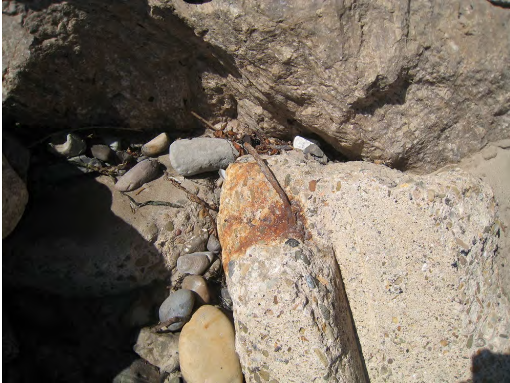
Concrete and rusted rebar in the Goleta Beach Park west end revetment.
