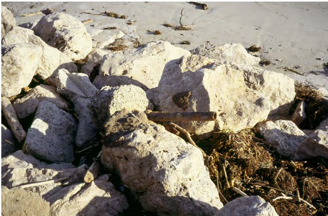
Debris and pipe in the Goleta Beach Park west end revetment. Concrete refuse is a significant fraction of revetment material.
