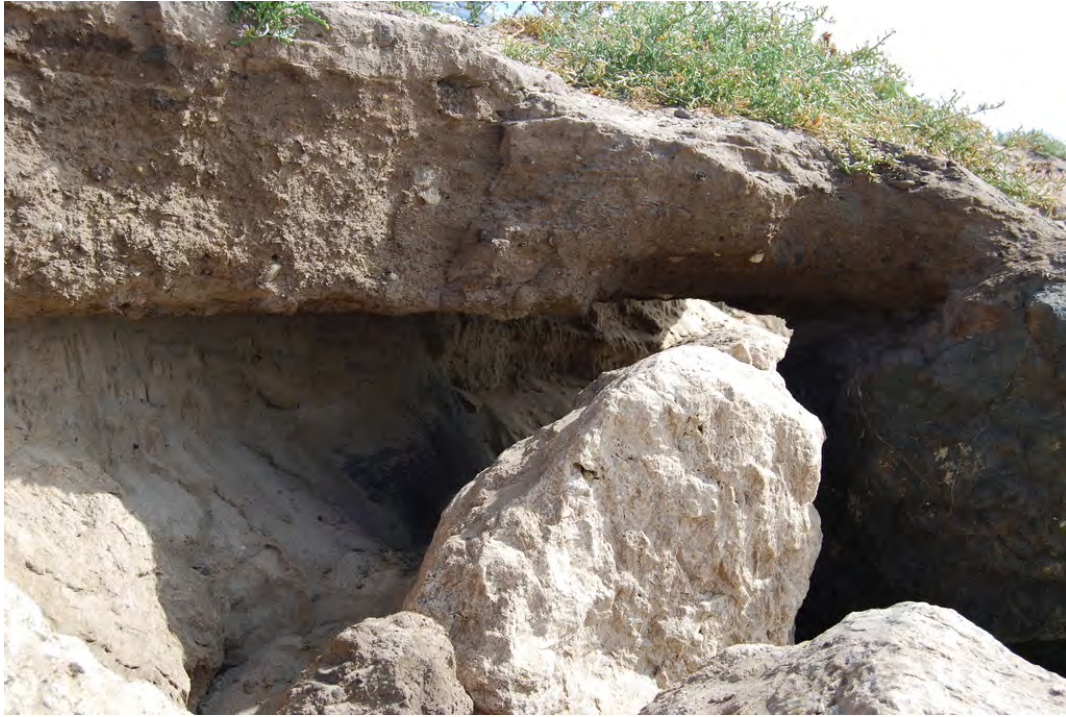
Revetment does not prevent erosion under parking lot 7.
