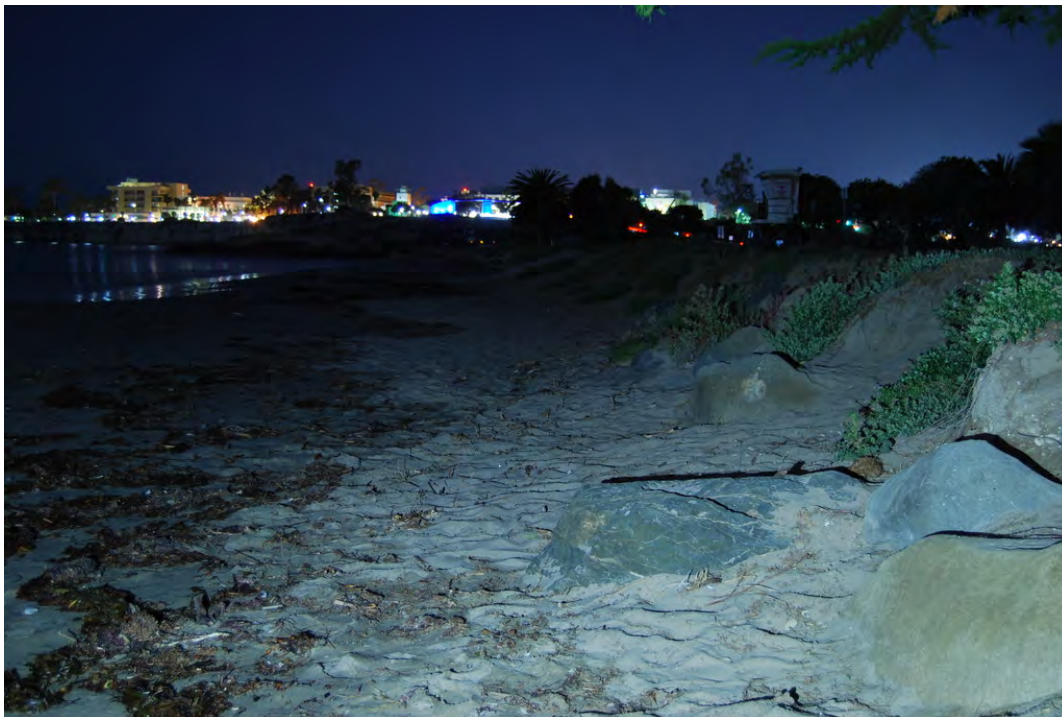
Goleta Beach mid-park revetment on May 4, 2015, at 10:46 PM. High water line following +5.5 ft high tide. EIR predicts no significant exposure before 2050. +6.3 ft tide due this Sunday, May 17, at 9:44 PM.
