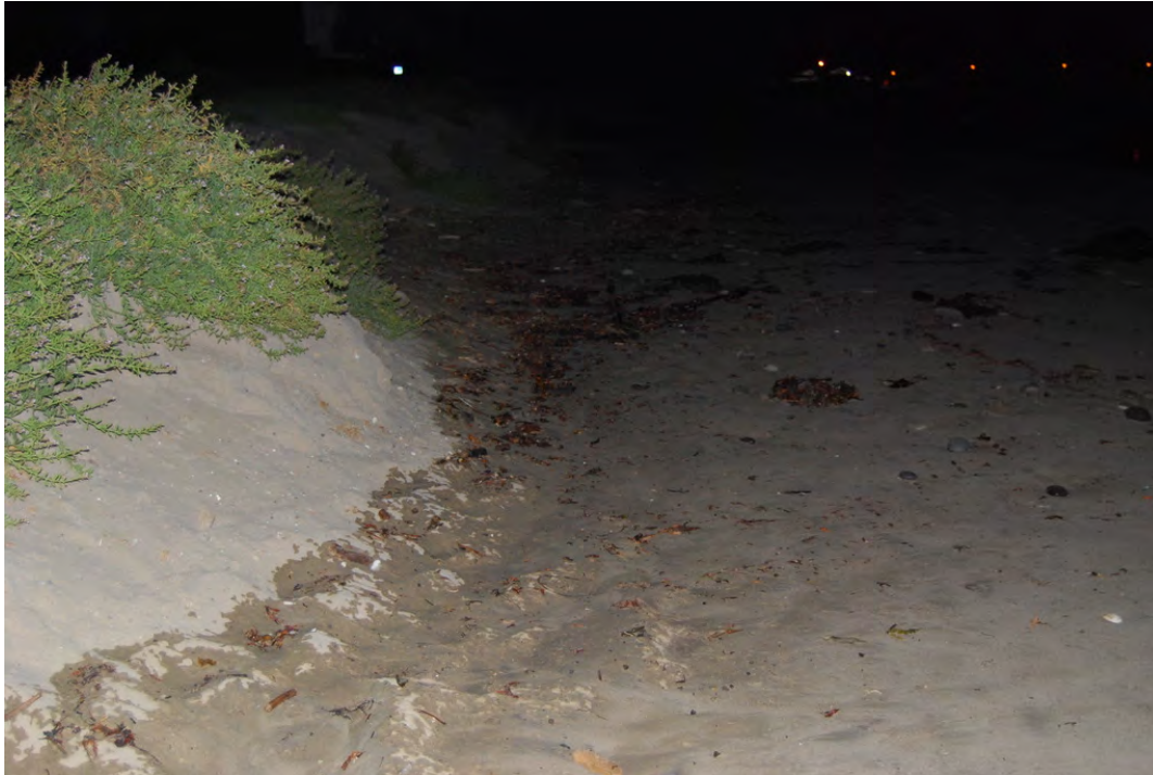
Goleta Beach mid-park revetment on May 5, 2015, at 12:08 AM. High water line at toe of buried rock following +5.5 ft high tide.
