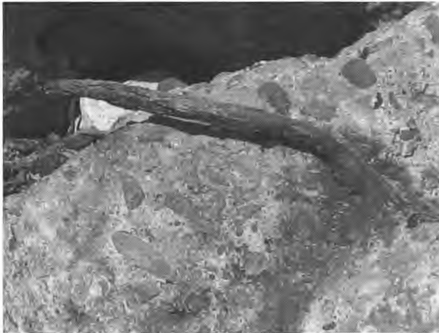
Photo 4. Close up of rebar in Goleta Beach rock revetment seawall. Everett Lipman. March 17, 2014.
