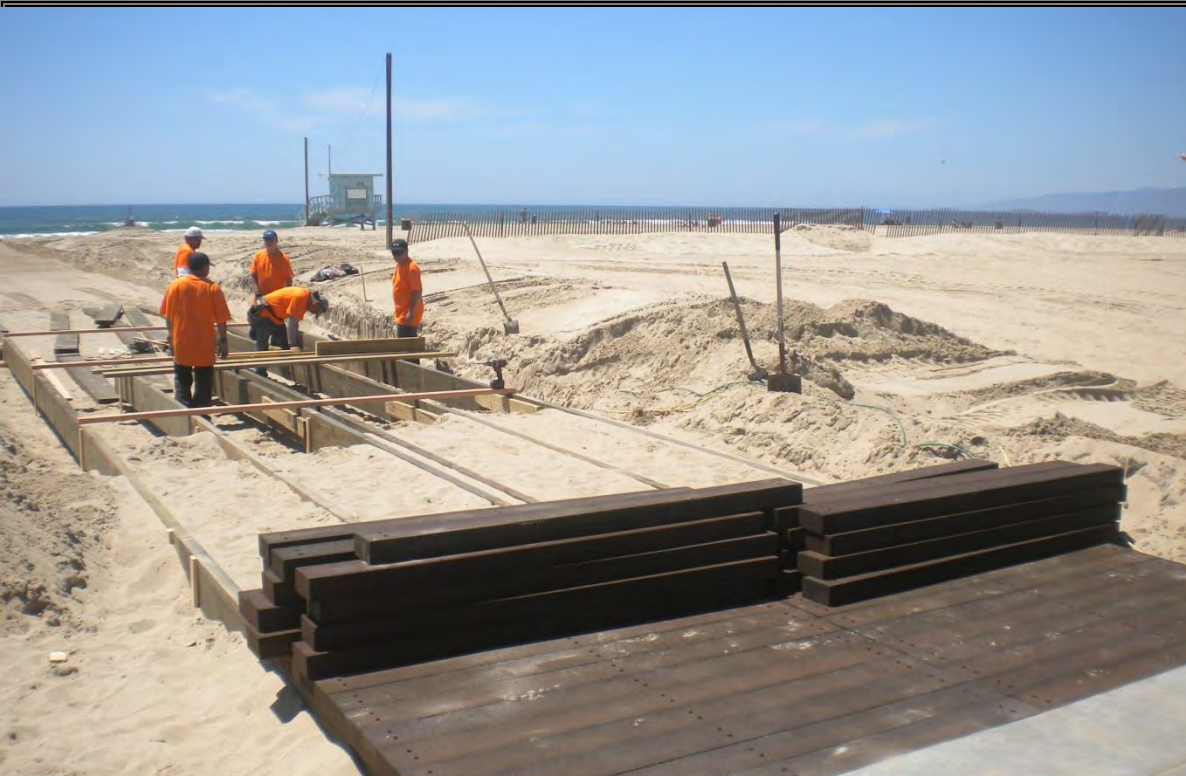
Example of Construction of Walkway Using Trex Planks
