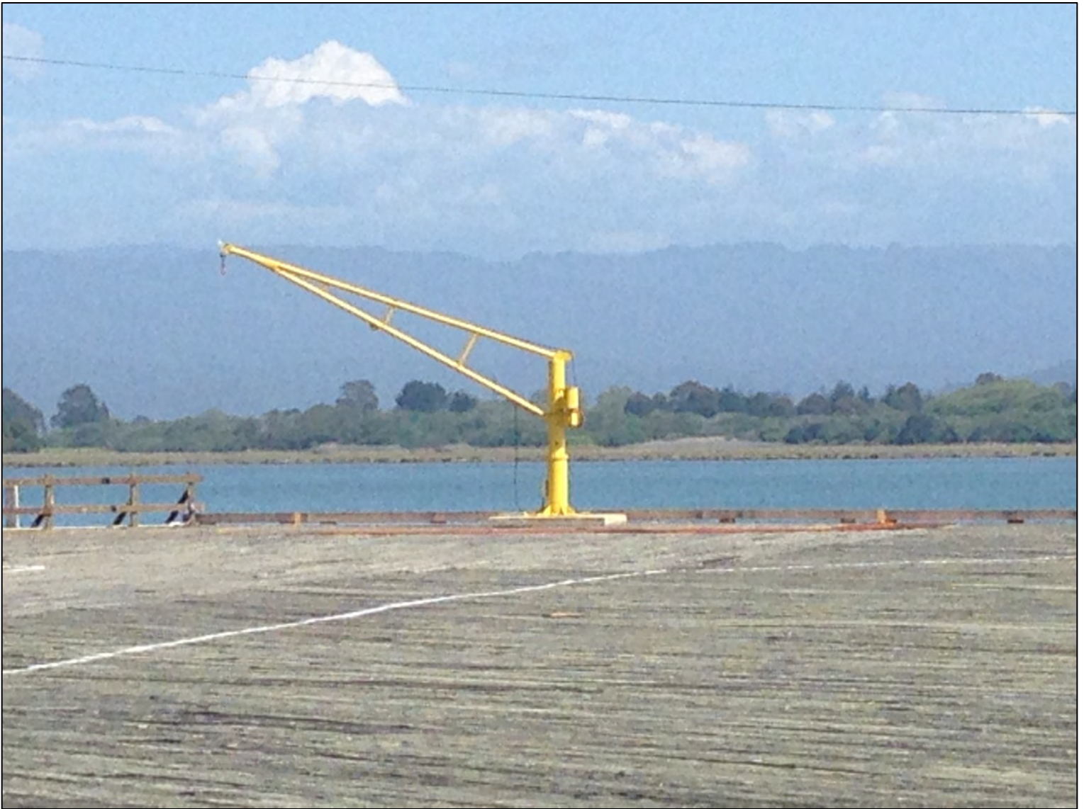
Photo 3. The proposed fish hoist that has already been installed without the benefit of a CDP.
