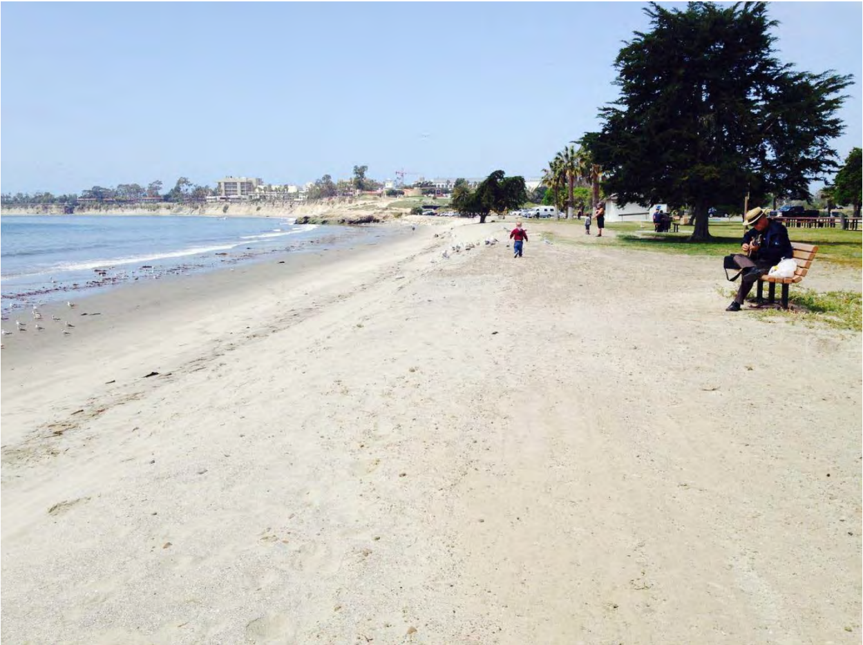
The above photograph was taken in April of 2016 and shows the park after the repairs occurred.
