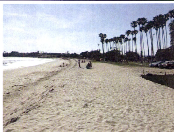
Repairs at Goleta Beach Park have been completed and lie buried beneath the sand (April 2016).
