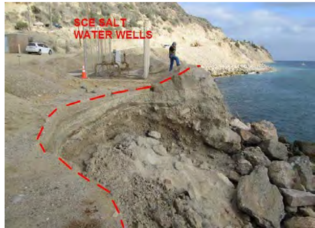
Photo 3: Erosion at East Side of Wells (Aug. 2015)
