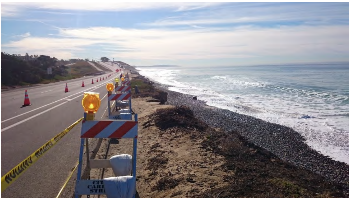
The photo above shows one of the locations along PCH where erosion is occurring. Emergency permits allowed rock protection for the winter months. Photo provided by San Diego Staff.
