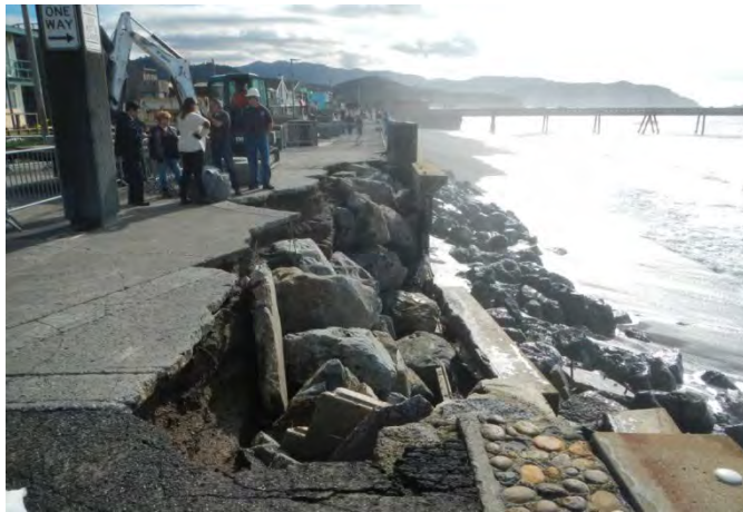
The photo on the left looks south at damage on Beach Boulevard, near the Pier in Pacifica. Wave overtopping caused erosion and loss of back fill material behind the seawall, resulting in a localized wall collapse and deep scour hole inland of the wall. Photos provided by North Central Staff.
