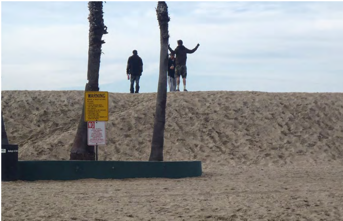
The photo above shows the beach berm constructed at Seal Beach to protect the inland development from flooding. The berm will be removed prior to the summer tourist season. Photo provided by Technical Services..
